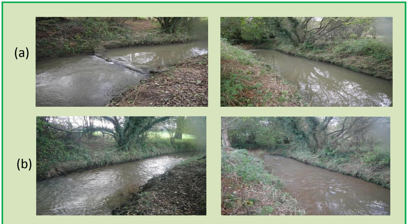
Figure 3; Section of Sussex Ouse showing ponded, homogenous habitat before (a) and after (b) weir removal and riffle installation ©Andy Thomas
