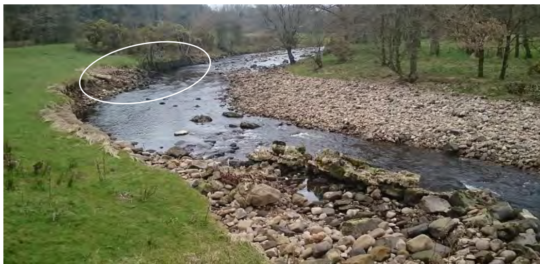
Fig 7. The uppermost section visited at Corless Mill where the mill leat infrastructure has been eroded into the river. Gabions are present u/s (white ellipse) but are only exacerbating erosion immediately d/s where there is insufficient root structure in the soils due to livestock access to the very bank top (see Fig 8).
