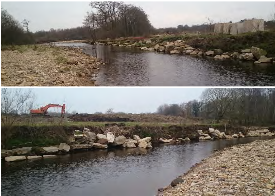
Fig 21. Introduction of boulder and concrete blocks to prevent erosion of the RB. See reference to video on page 9.
