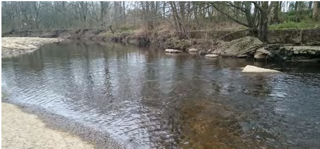
Fig 15. Looking d/s from the dilapidated weir (concrete bottom left & top right of shot). Without the diversion of the weir, the river is now cutting a more natural curve into the RB.
