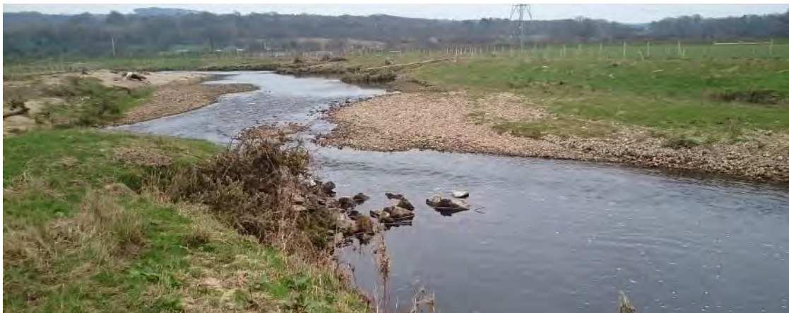
Fig 29. Looking u/s at channel variability instigated by artificial groynes to divert flow. Note tree planting on LB but lack of cover at the water edge.
