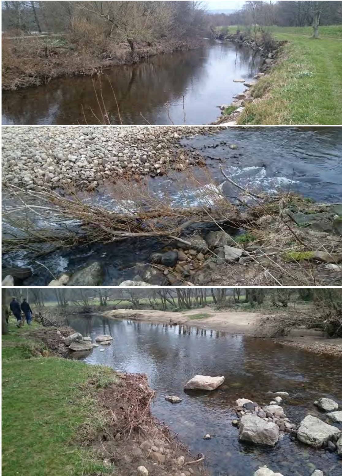
Fig 26. Examples of habitat management: upper panel looking u/s at mowed LB compared to relatively natural RB, note also the rock armouring of the LB; mid panel – fantastic laying of willow; lower panel looking d/s at scalloping of LB caused by boulder placements, and note erosion of mowed bank top.
