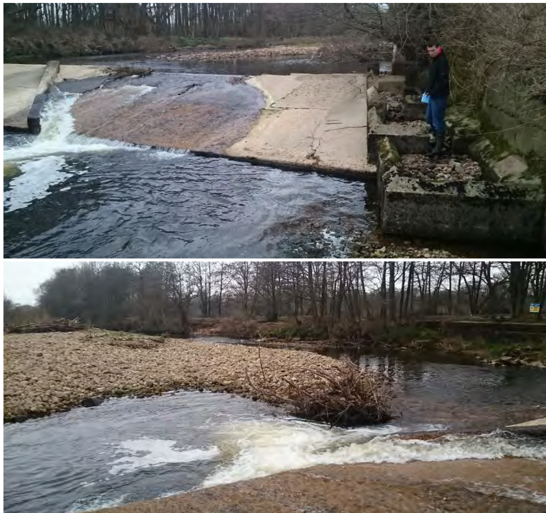
Fig 25. The weir next to Clevelymere: upper panel looking u/s at the damaged crest, baulk, and dry fish pass; lower panel d/s at the vast deposit of substrate.
