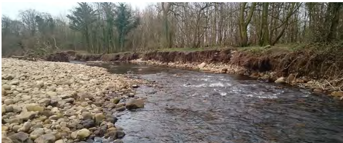
Fig 16. D/s from the dilapidated weir, the RB is subject to considerable erosion despite mature trees in the riparian zone because the full energy of the spate flow is directed there now the weir has gone.
