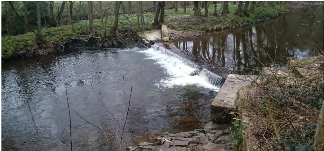
Fig 1. The defunct weir at Dolphinholme Farm is an obstruction to fish passage, causing impoundment and associated hydrogeomorphological issues u/s. The notch appears to be blocked by a single boulder and could be exploited.
