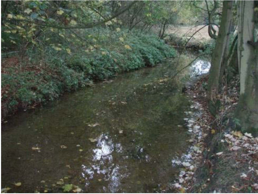
Photo 12 Accumulated sediment upstream of the structure creates a wide, shallow channel
