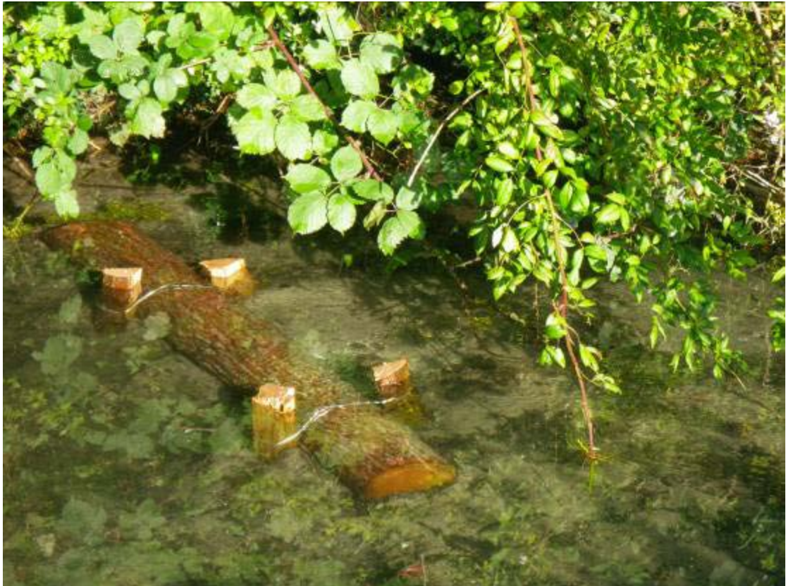
A freshly installed LWD deflector adjacent to some good overhead cover will create a good lie. The mid-channel end of the deflector points slightly upstream.
