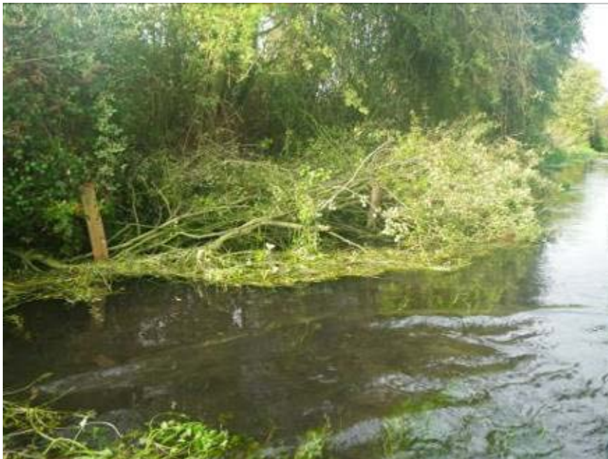
Brushings pegged into the margins to provide enhanced cover for juvenile trout on the upper Loddon
