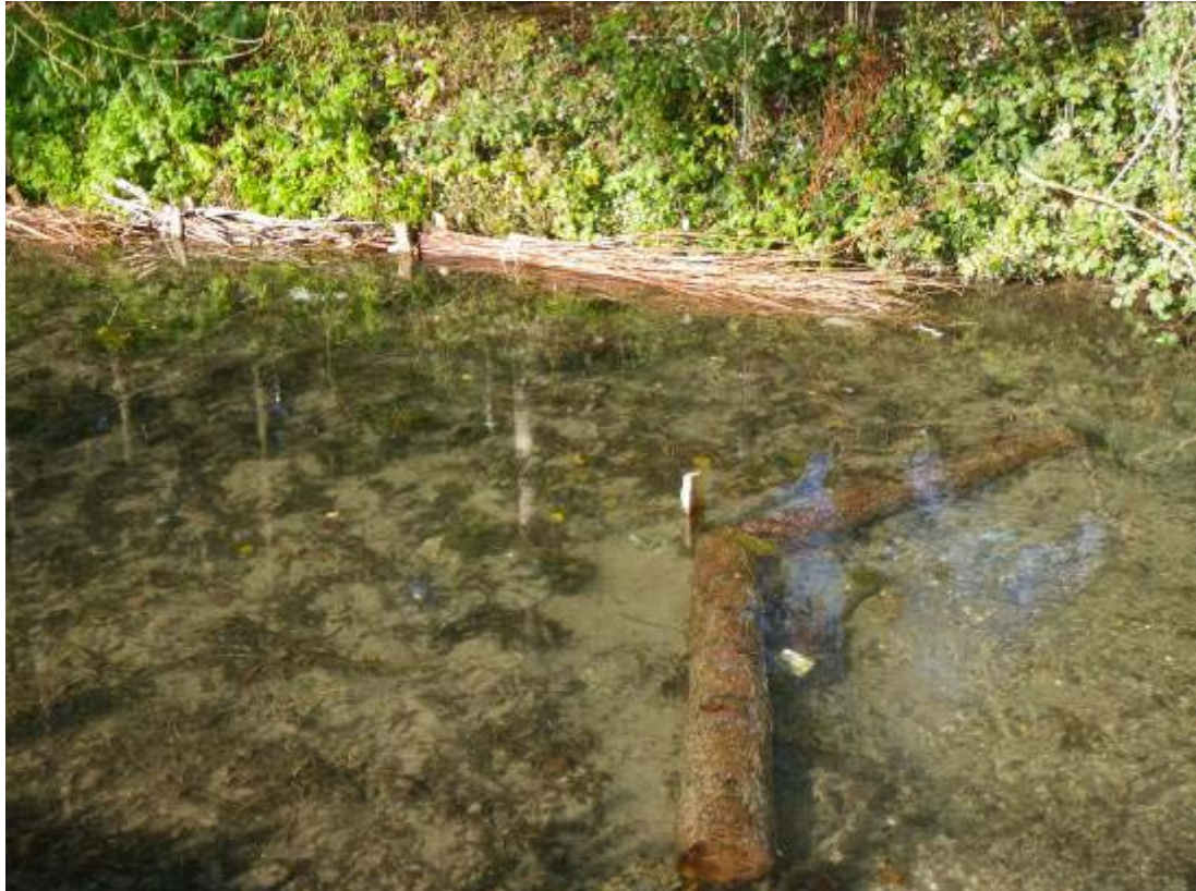
A small upstream "V" deflector designed to promote mid channel bed scour. Note the post designed to catch weed and provide cover.
