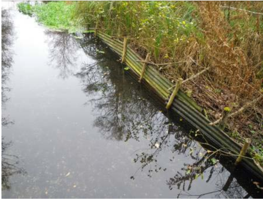
A short section of bank revetted with corrugated tin. A poor quality margin for plants, invertebrates and fish
