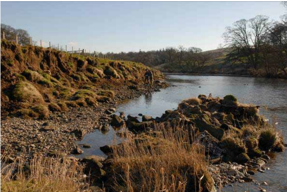
Proposed start (Island) of revetment works
