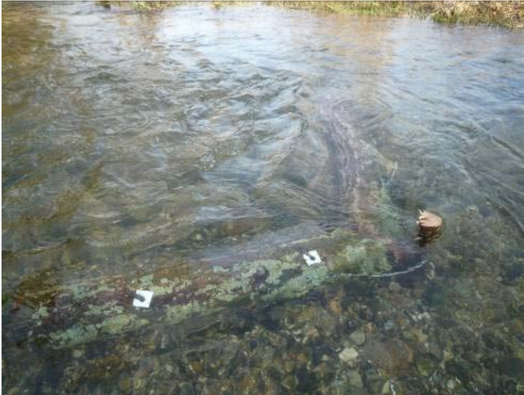
Two pieces of LWD configured to form an upstream "V". Structures like this scour local pots in the shallow bed and promote a clean, loose ramp of gravel downstream. A few of these on the top beat would promote better lies and improve spawning potential.
