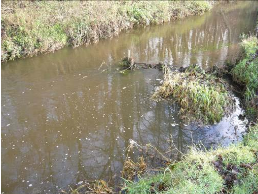
A post and chicken wire flow deflector. Deflectors pointing downstream can make the channel even wider
