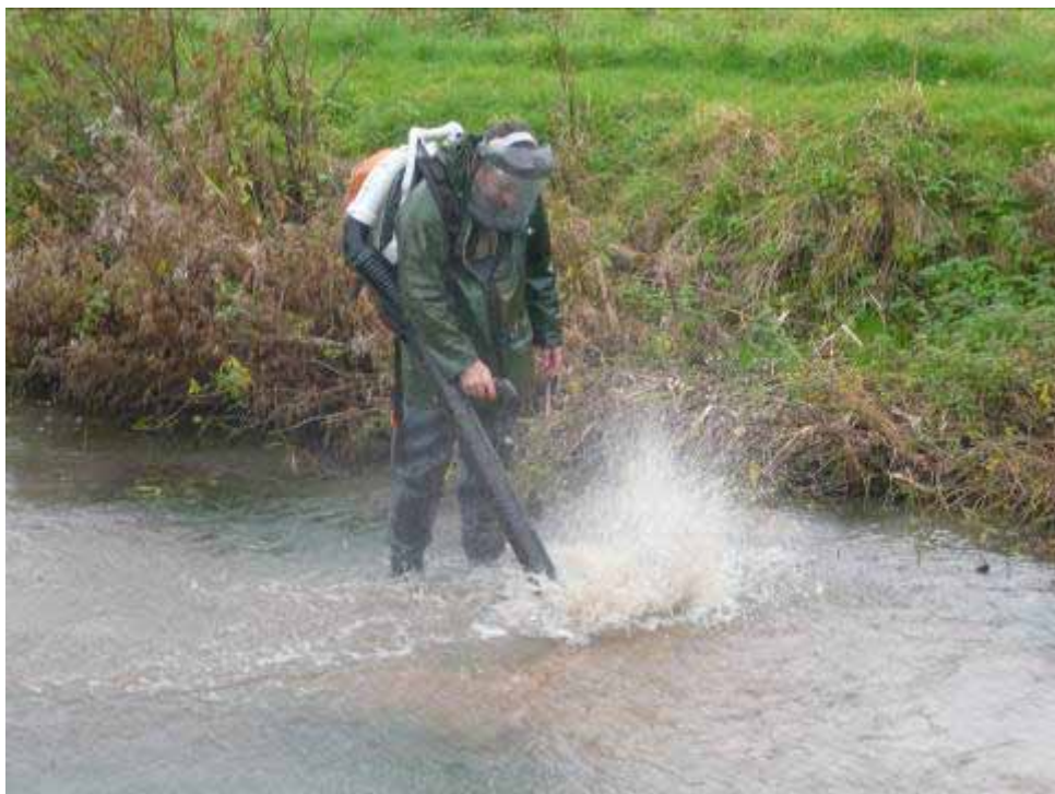
Gravel cleaning using a backpack leaf blower.
