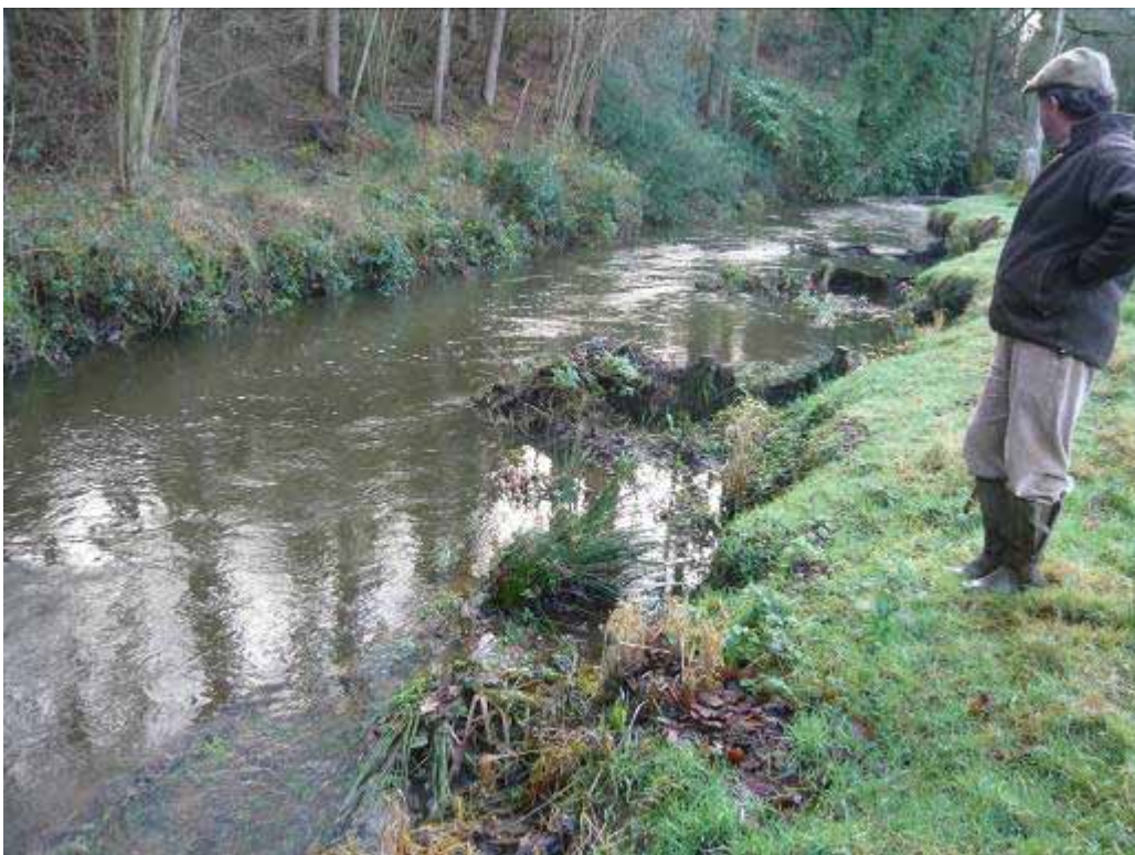
A series of chicken wire groynes. Some habitat has been created but better results can be achieved with tree trunk deflectors.
