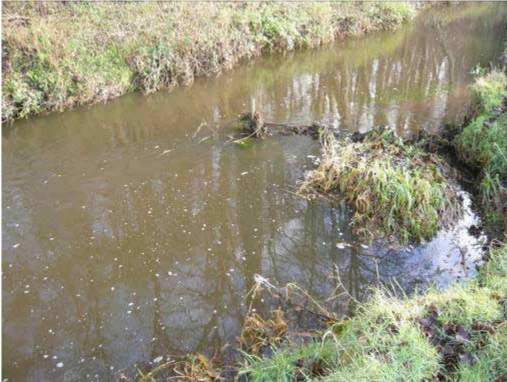
A post and chicken wire flow deflector. Deflectors pointing downstream can make the channel even wider
