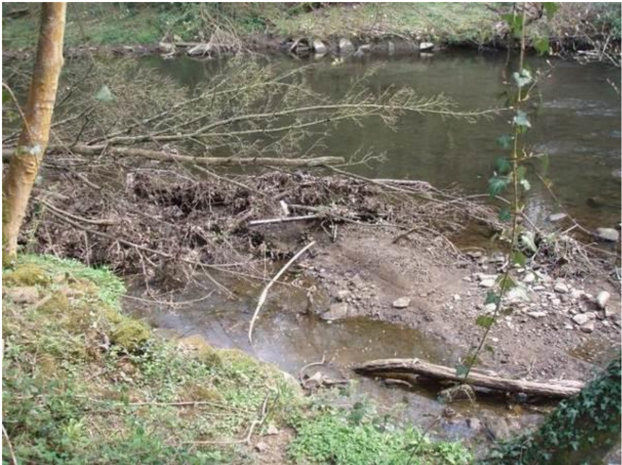
Figure 17. A perfect example of how a tree kicker can be employed to create deposition in the river margin that will focus flows down the far side of the channel.
