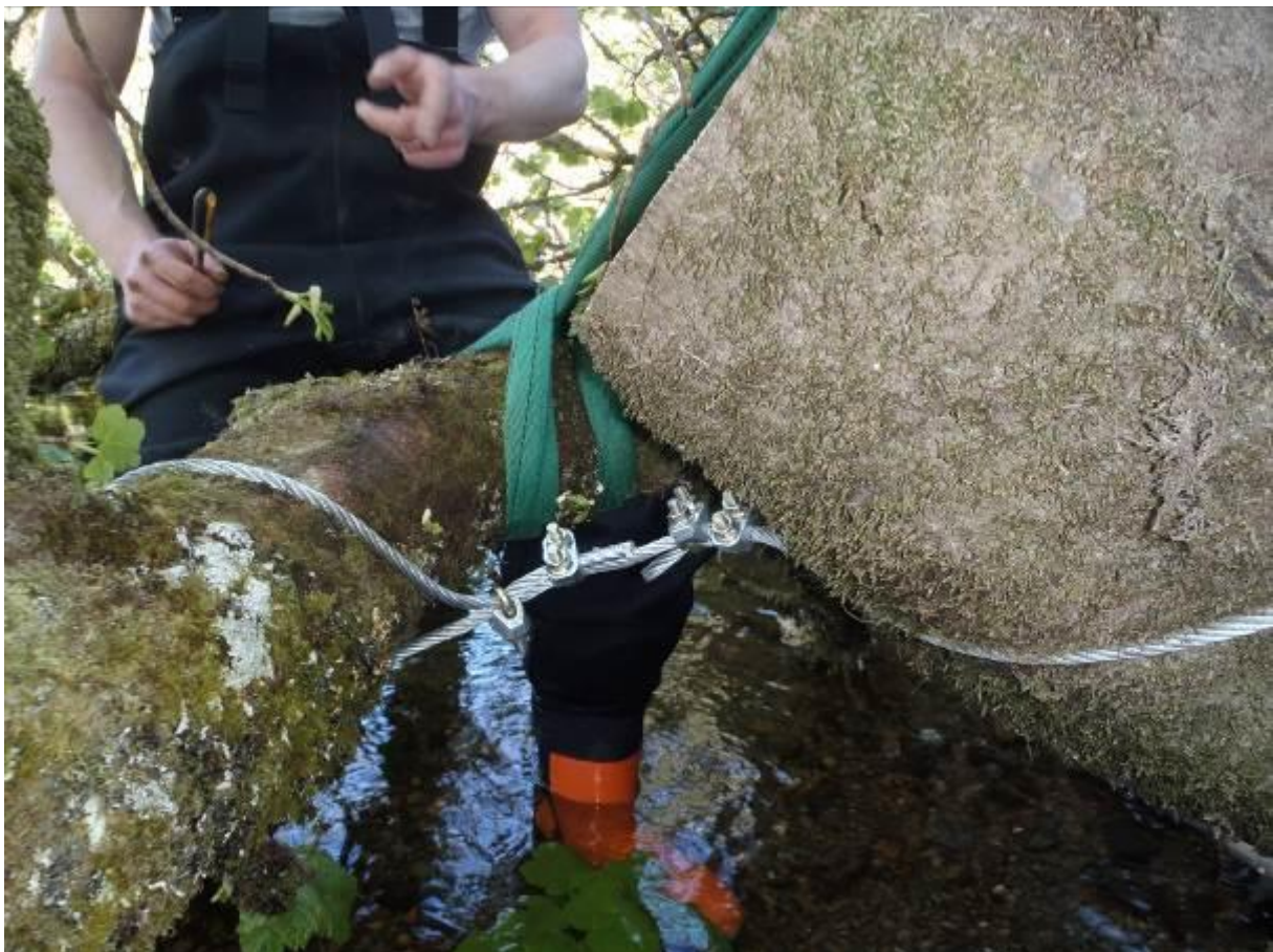
Figure 16. A basic tree kicker cable setup using 4000 kg breaking strain cable and two sets of cable clamps. The webbing strap in the background is used to pull the kicker close to the stump for fastening but is removed once the cable is fully fixed in place.
