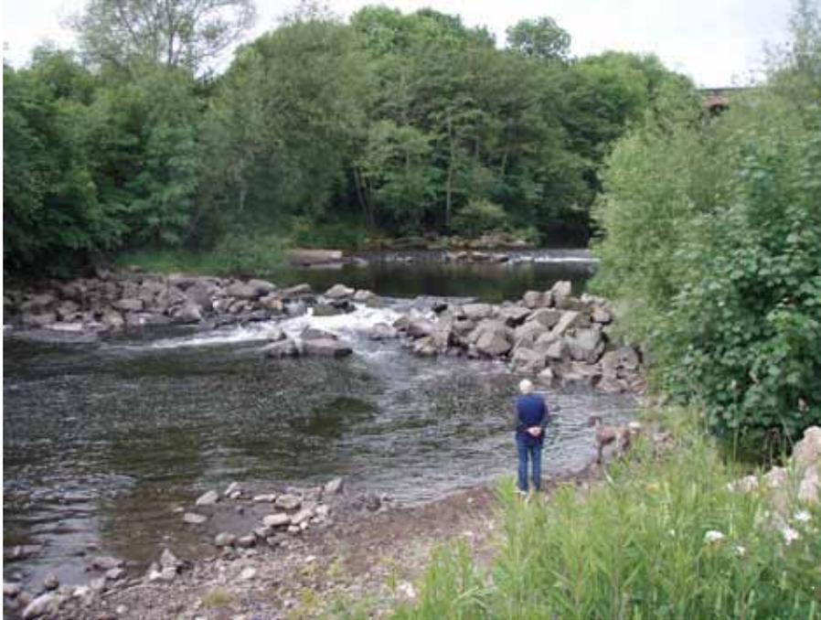
Photo 1 Weir and ford (background) and block stone pre-barrage downstream of Witton Park viaduct
