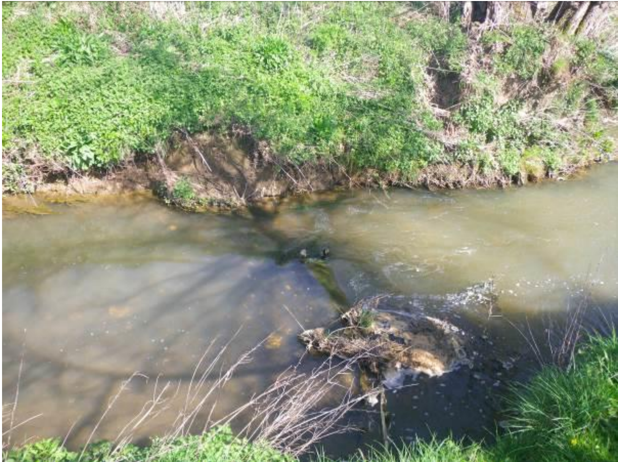
Photo 3. Woody debris groyne promoting useful bed scour.
