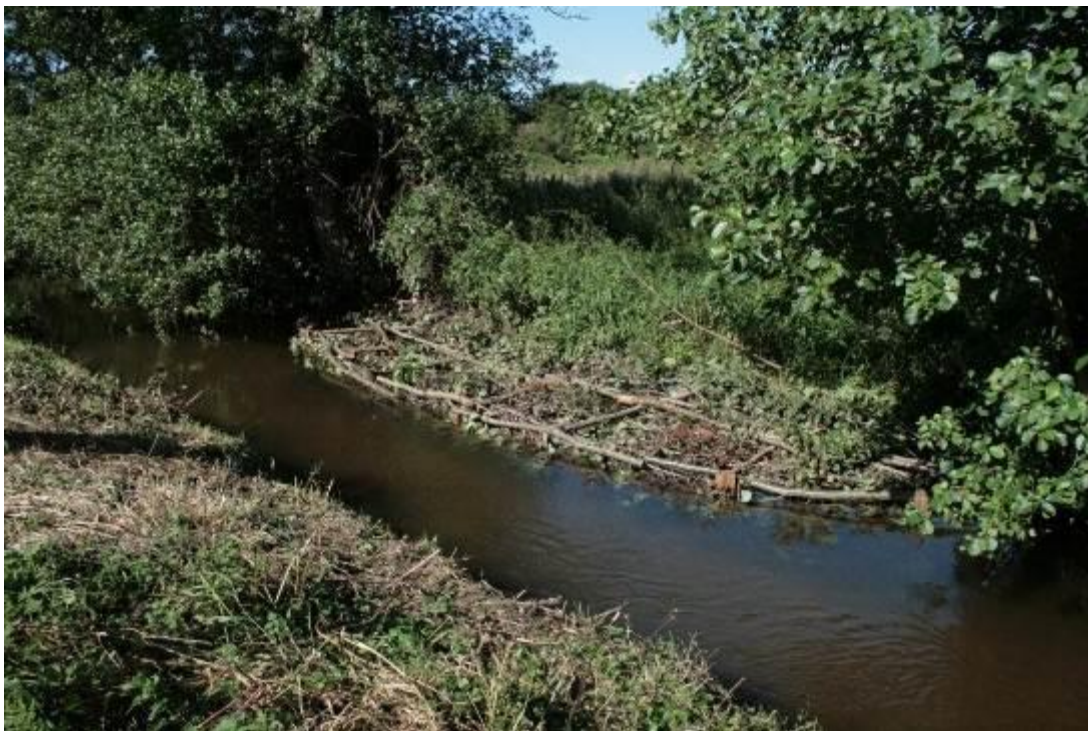
Photo 7. An example of a brushwood shelf on the River Glaven, Norfolk.
