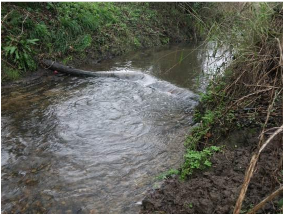
Photo 6. An upstream facing V structure with narrow gap made from two separate logs which concentrate the flow and reducing risks associated with upstream deposition.
