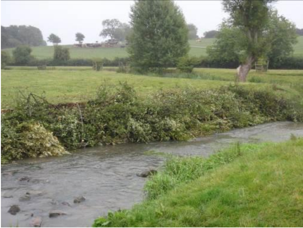
Photo 8. Brushwood packed against the face of an eroding bank on the Great Ouse.
