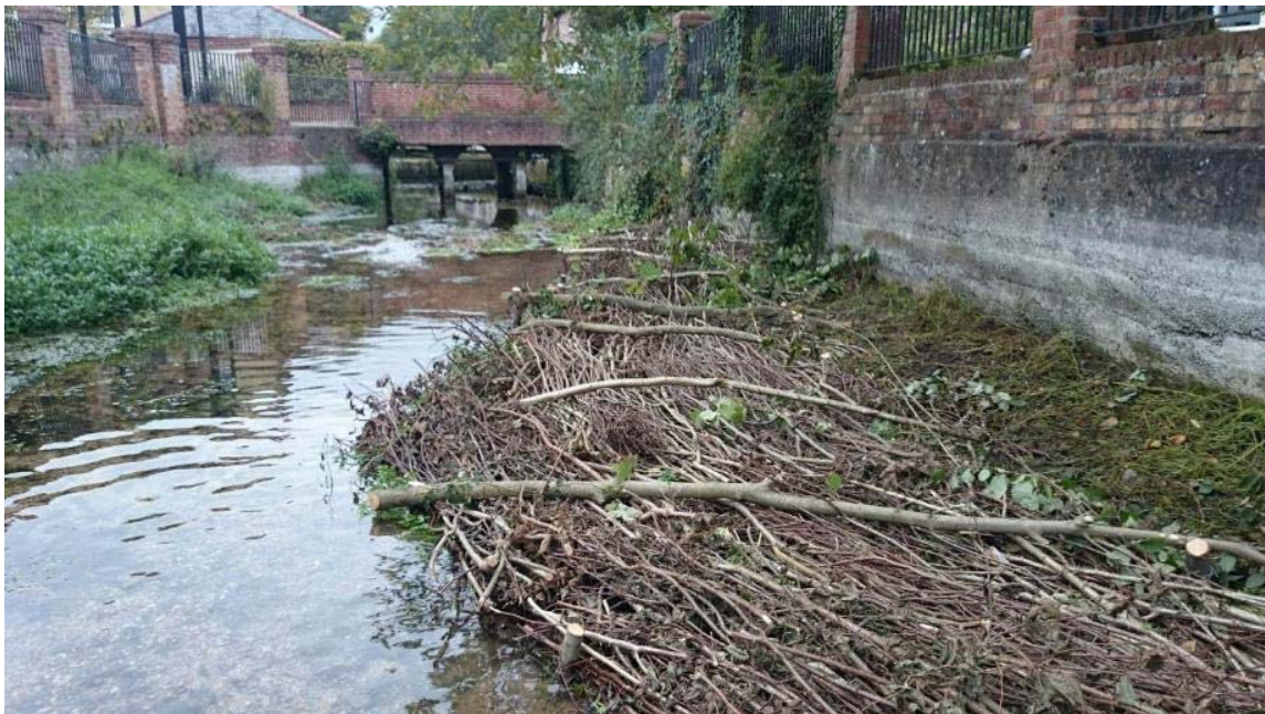
Photo 14 Marginal ledges made from stakes, battens and packed with brushwood could be used to achieve a similar channel narrowing effect, in addition to providing good crayfish habitat.
