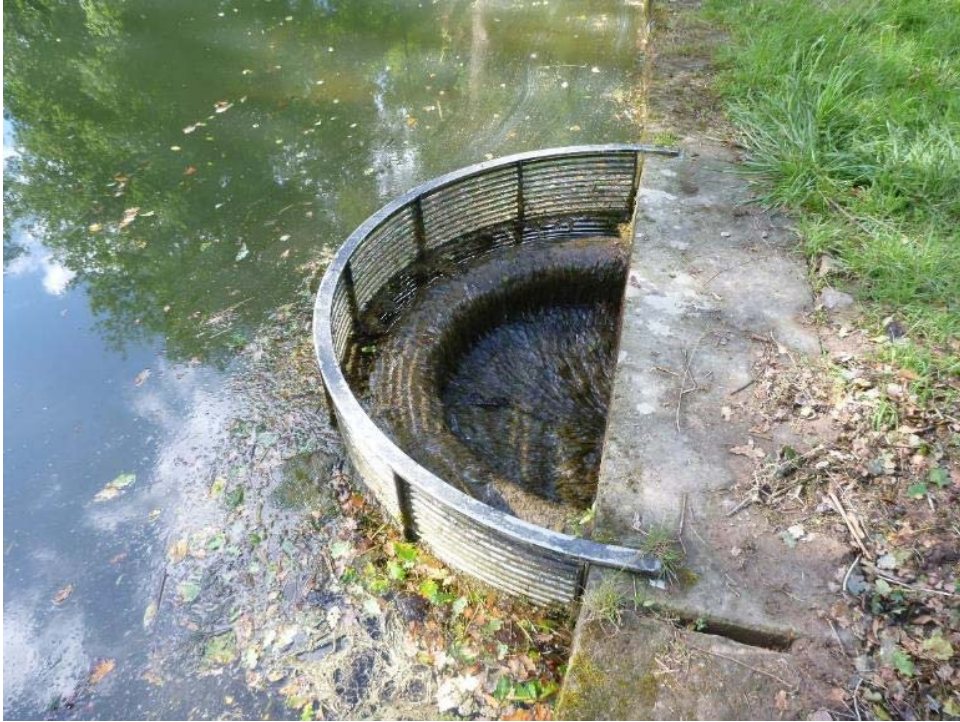
Photo 4 The outflow from the restored pond. There is also a restored ram pump at the southern end of the dam.
