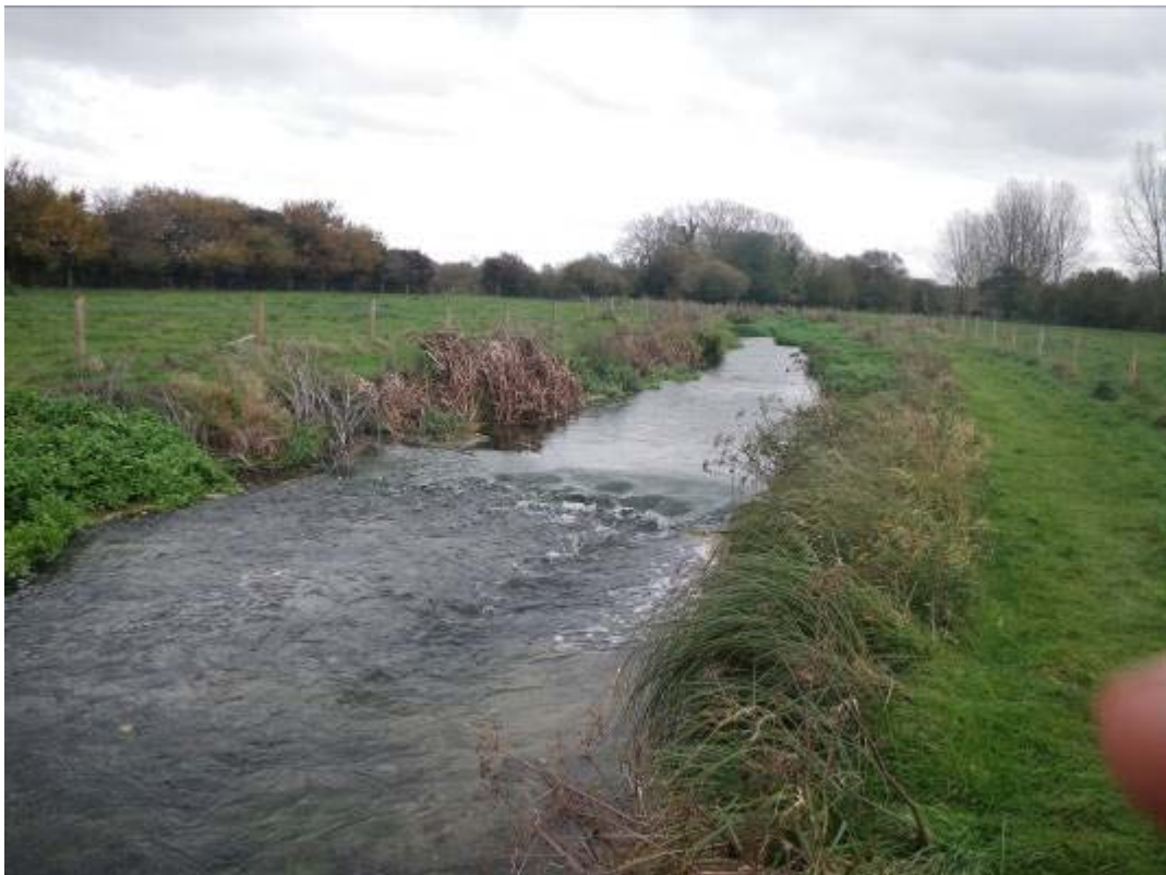
The remains of a collapsed stone weir providing some variation in channel form.
