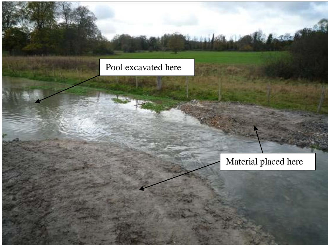
"Dig and dump" employed on the River Meon to promote "pool riffle" habitat
