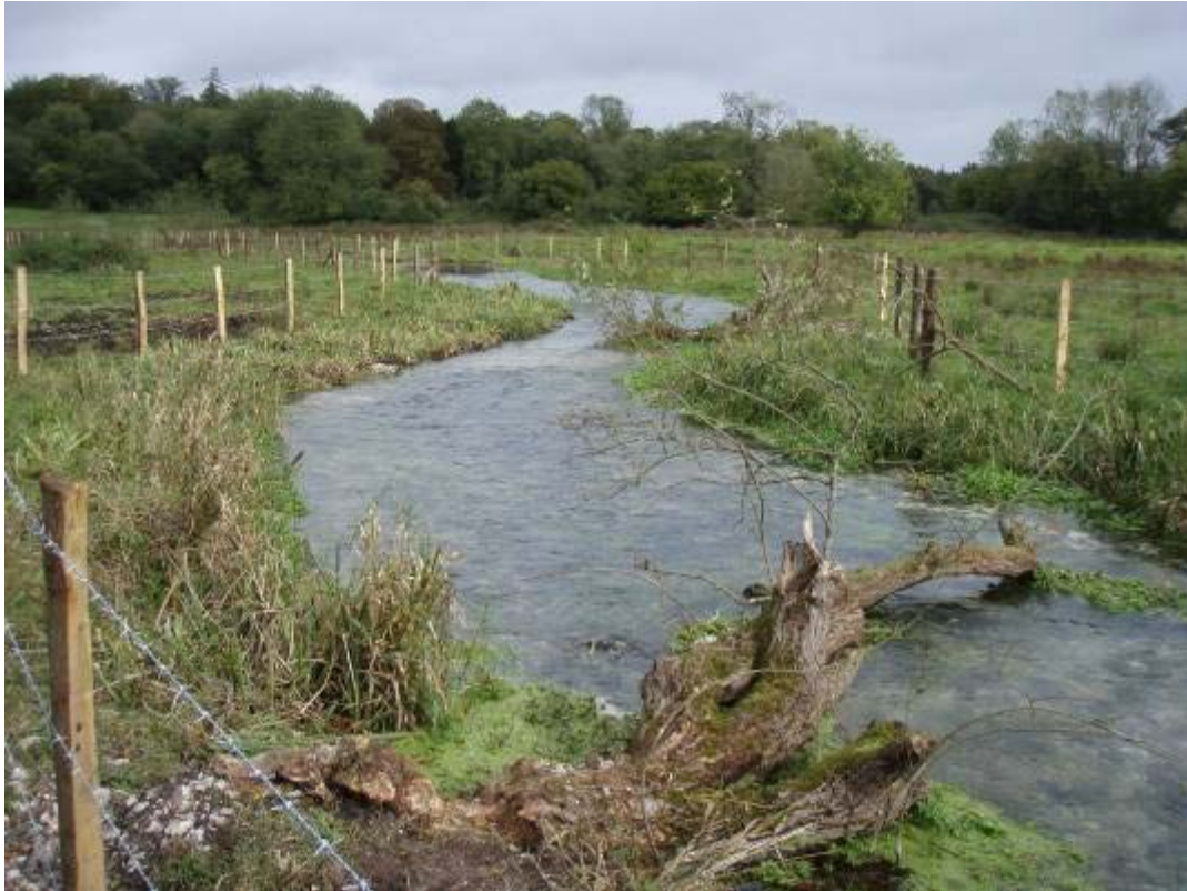
A newly planted "live willow" deflector placed into the upper Itchen to promote local bed scour
