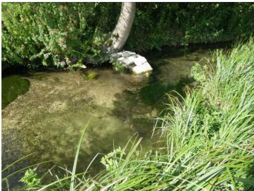
Bag-work flow deflector packed under an overhanging ash tree.
