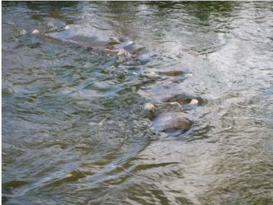
A large tree trunk deflector pegged into the Oakley Stream on the Test used to improve gravel quality for spawning.
