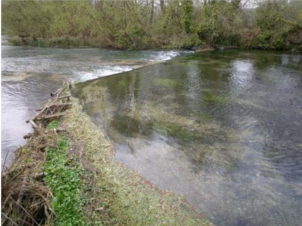
The low V weir where the bed has regraded upstream. Not an impediment to fish migration but a restriction on habitat development upstream. Note the presence of the red non-native plant Azolla in the foreground.
