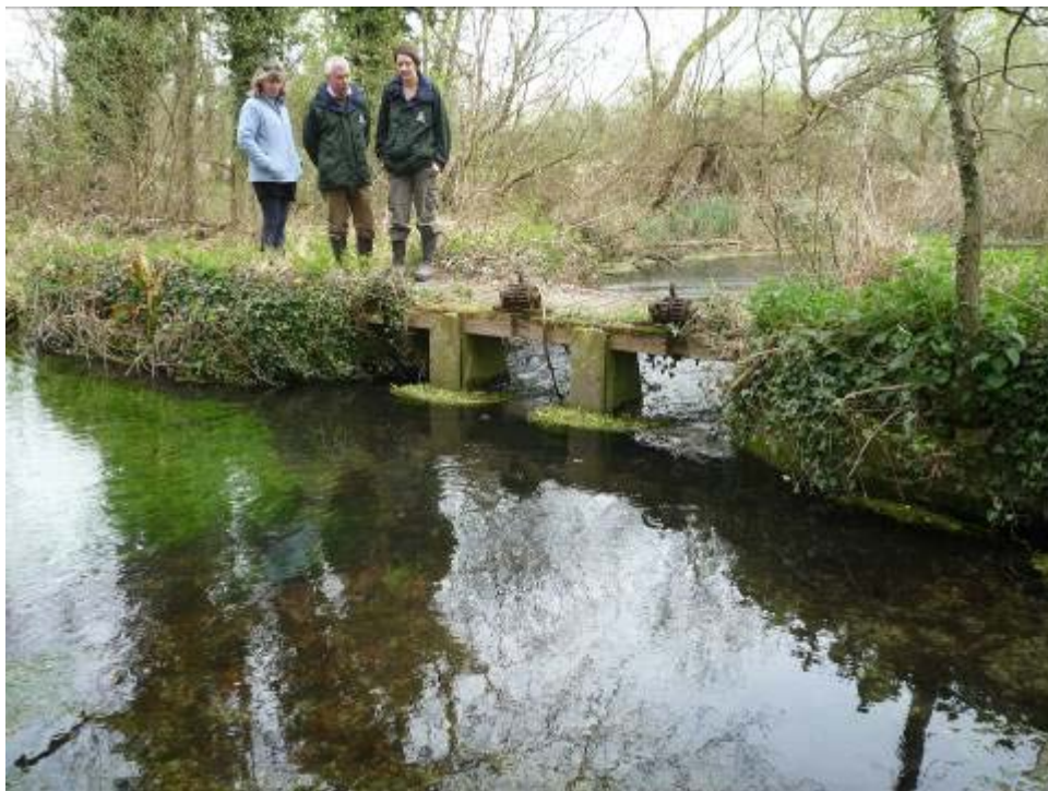
Bottom hatch which lends itself to being bypassed with a cut-through channel
