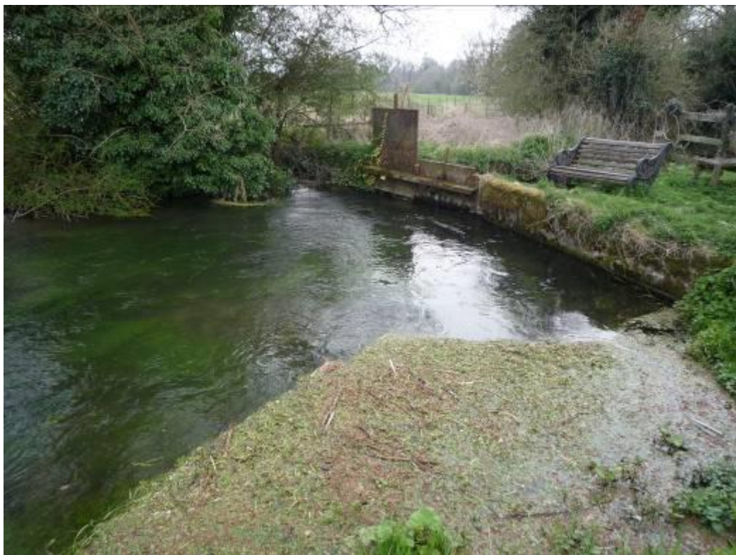
Middle hatch on the top main river beat with one gate drawn.
