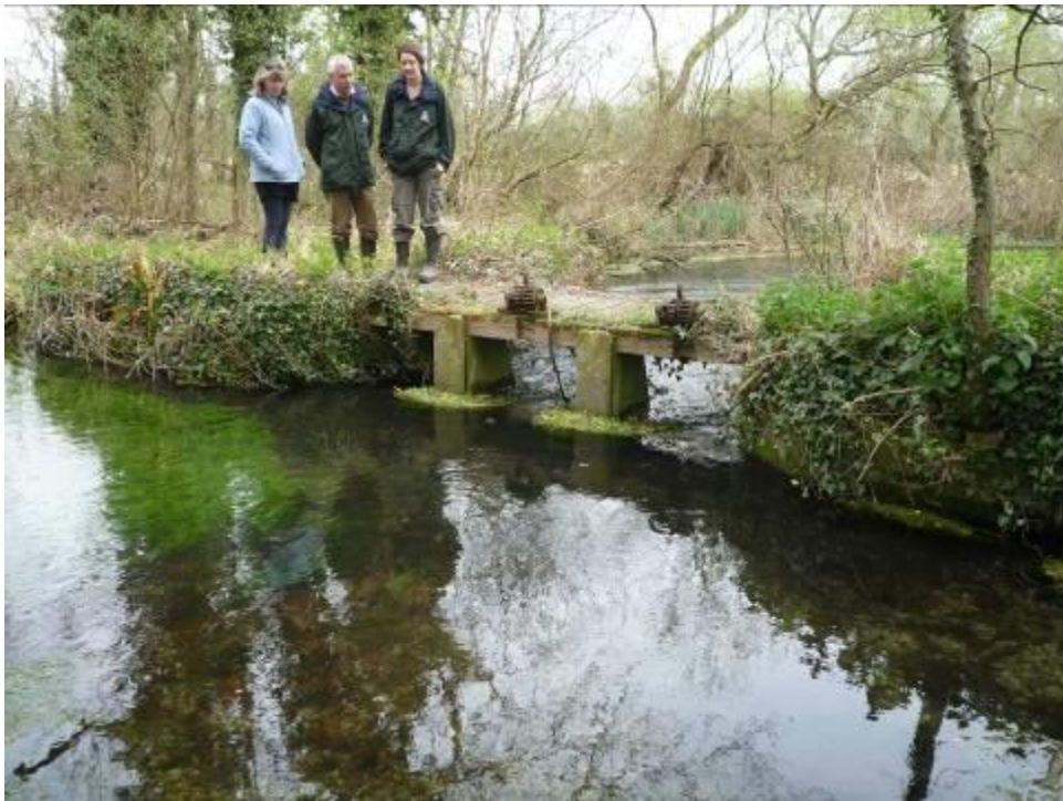
Bottom hatch which lends itself to being bypassed with a cut-through channel
