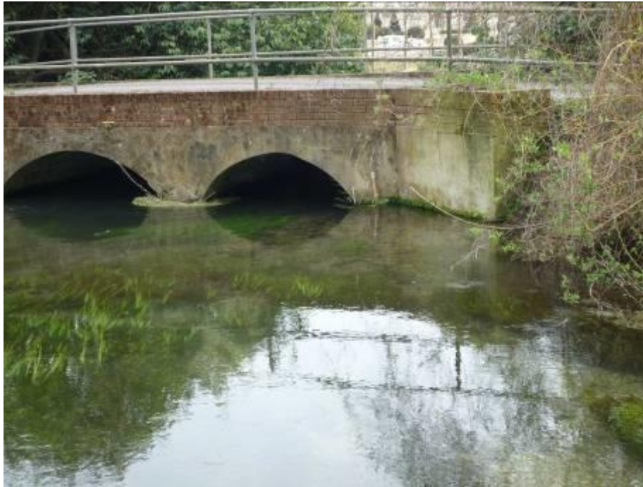
Road bridge at the bottom boundary. Lowering the bed level beneath the right hand arch should promote increased velocities in the bottom of the carrier
