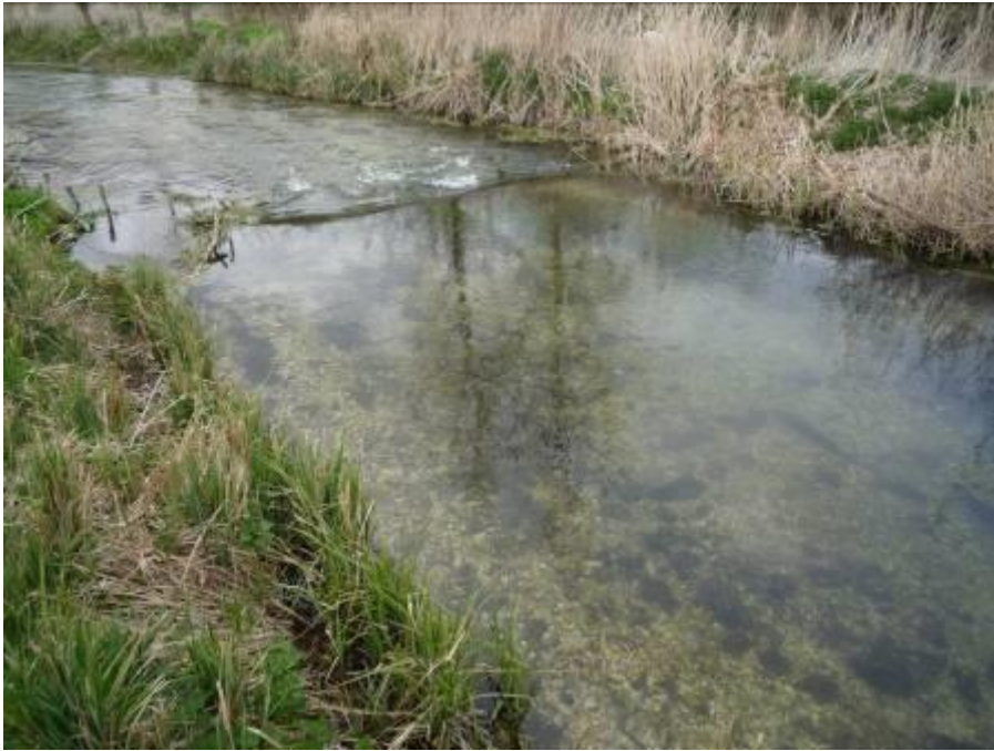
A small weir which looks to have been installed for fishery purposes. A half weir created by pegging in a tree trunk would be a better option
