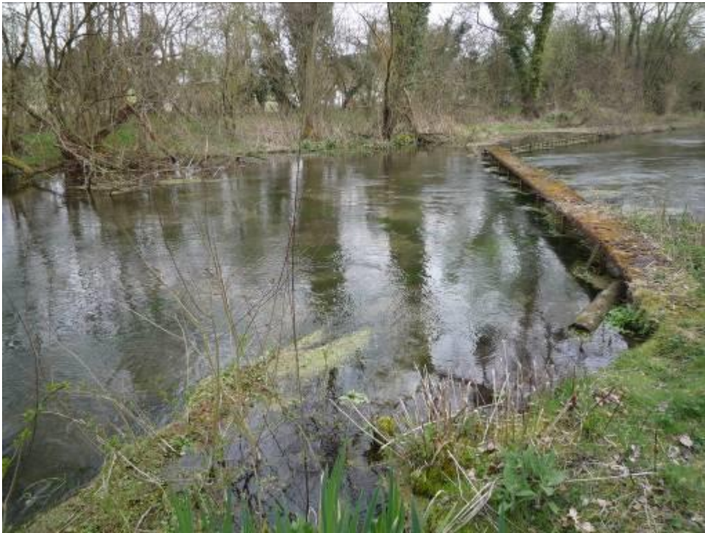
Old metal walkway and stantions near the bottom boundary can catch cut weed and impound water velocities on the main beat
