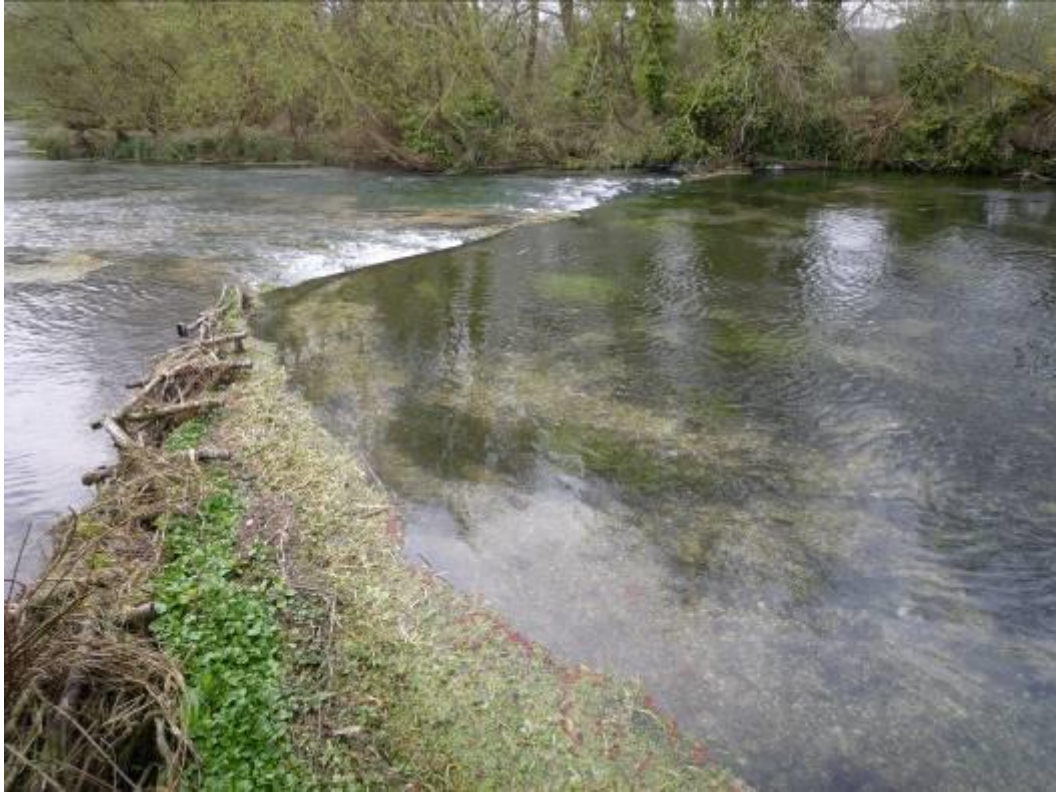
The low V weir where the bed has regraded upstream. Not an impediment to fish migration but a restriction on habitat development upstream. Note the presence of the red non-native plant Azolla in the foreground.
