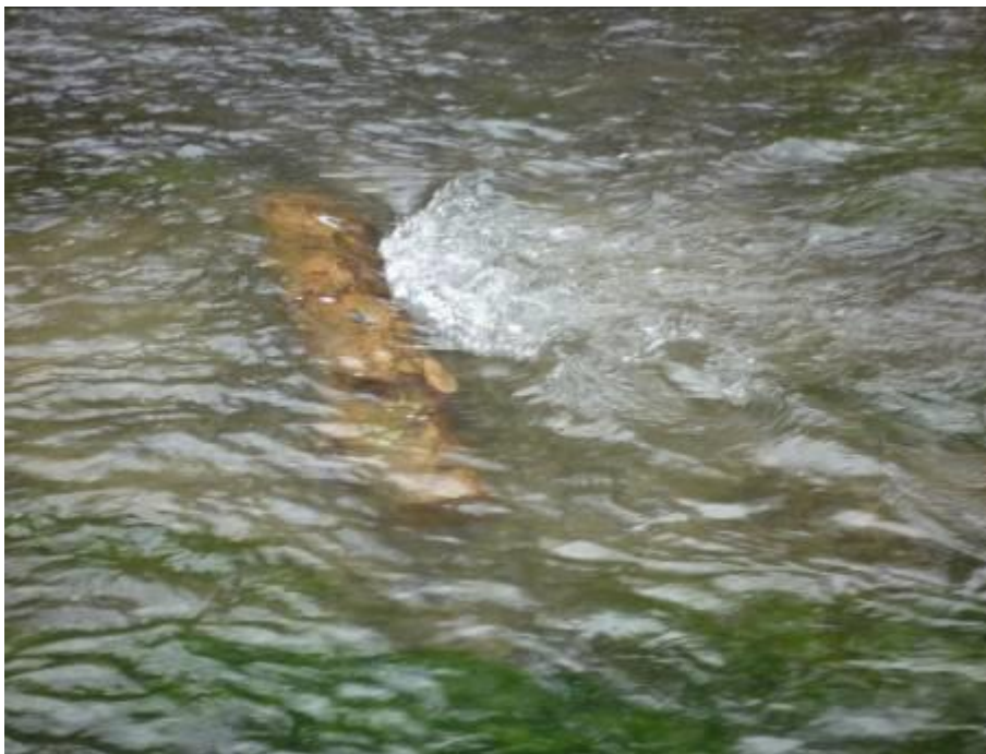
An example of a piece of LWD used to promote local scour on a riffle and promote enhanced spawning habitat
