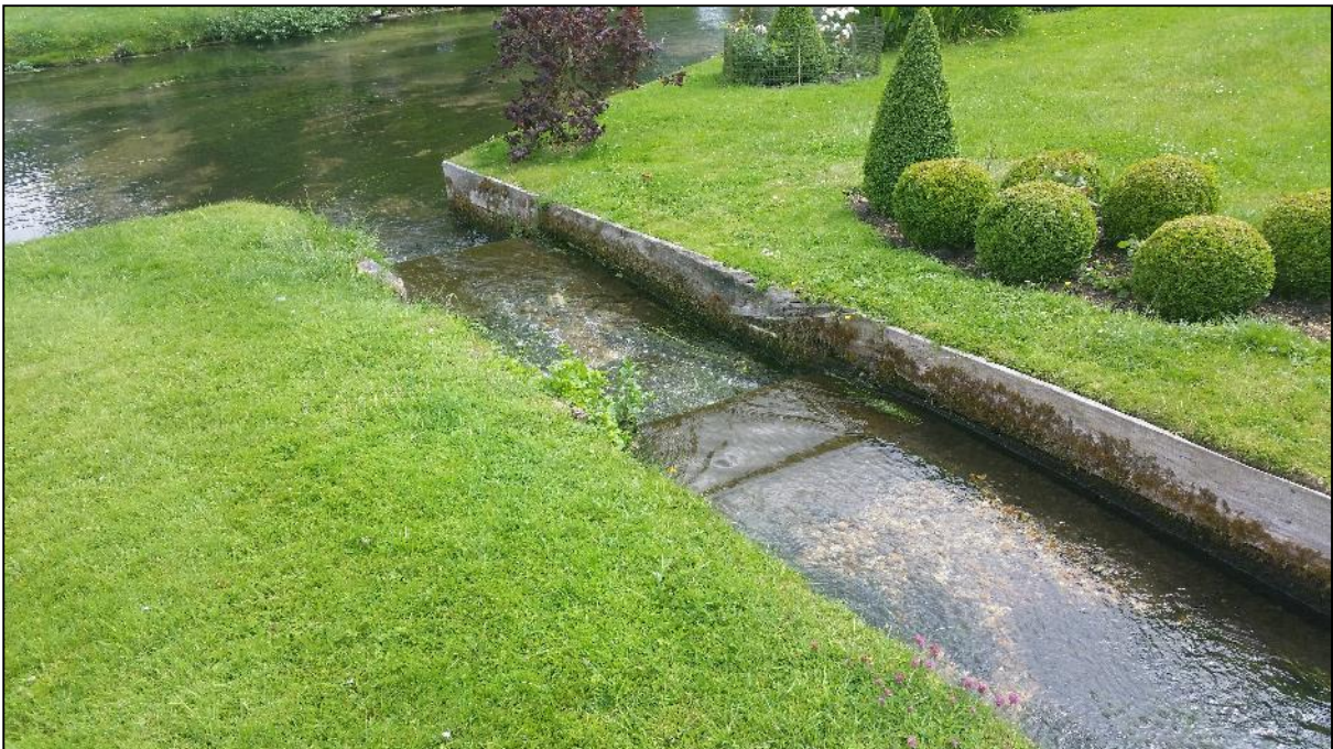
Figure 16: Shuttering and concrete weirs limit habitat quality at the confluence
