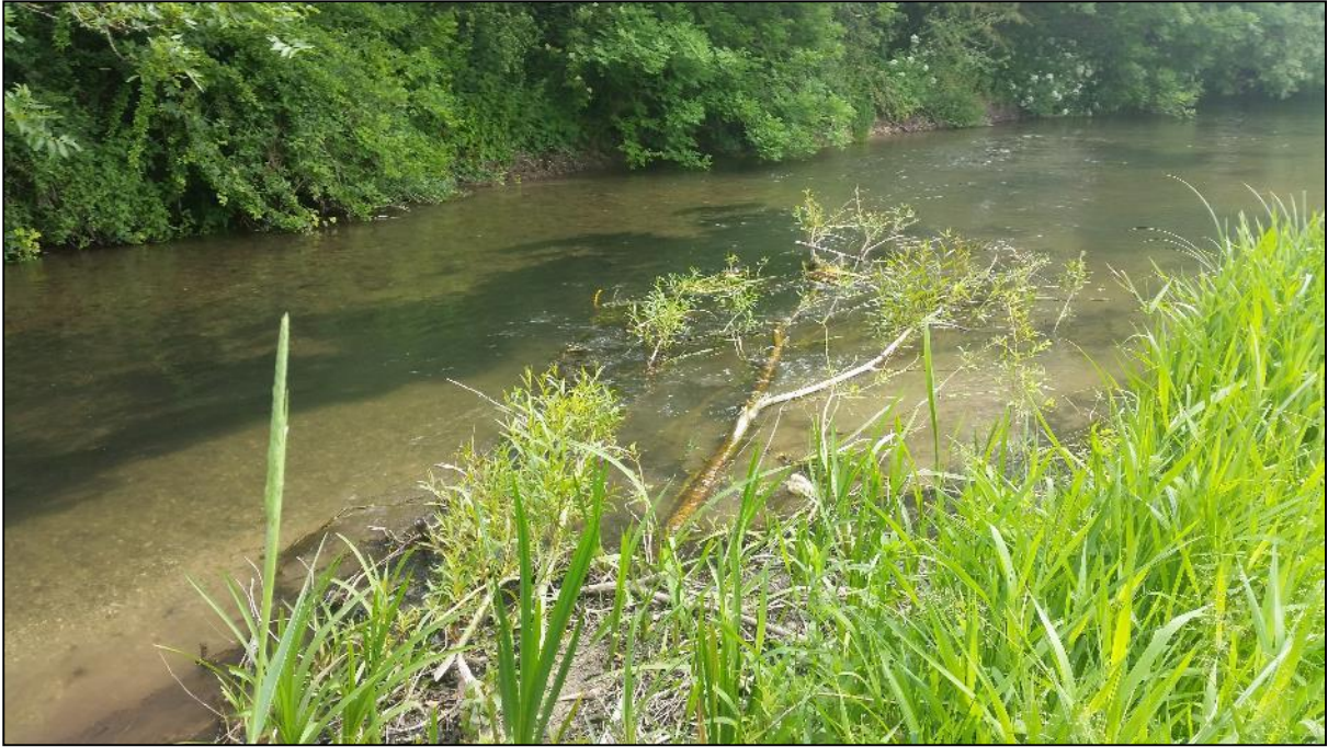
Figure 18: An example of a hinged live willow diversifying flows and providing excellent cover and fish refuge
