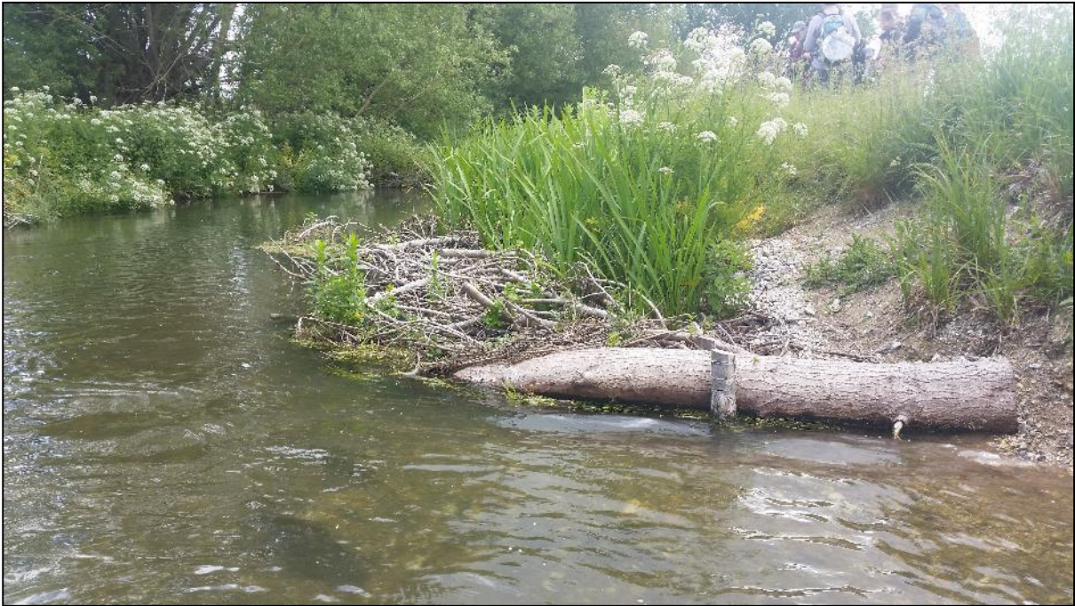
Figure 17: A log and brushwood berm installed on the Hampshire Avon has become colonised with iris ( Iris pseudacorus )
