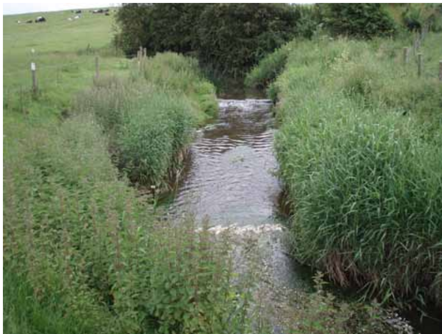
Photo 8 Low weir constructed to supply head for running incubation box
