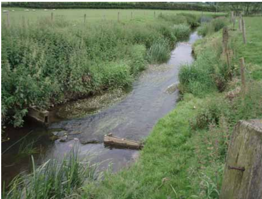
Photo 6 Flow variation created by paired deflectors and bricks, promoting growth of Ranunculus sp. and deterring emergent vegetation
