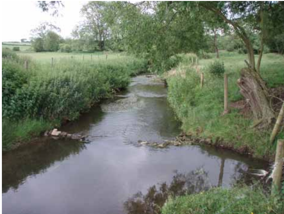
Photo 7 Area cleared of emergent vegetation where eight tonnes of gravel was introduced along with four sets of flow deflectors
