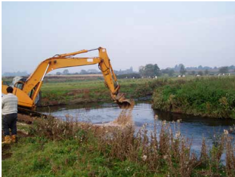
Photo 9 Reintroducing gravel riffles
