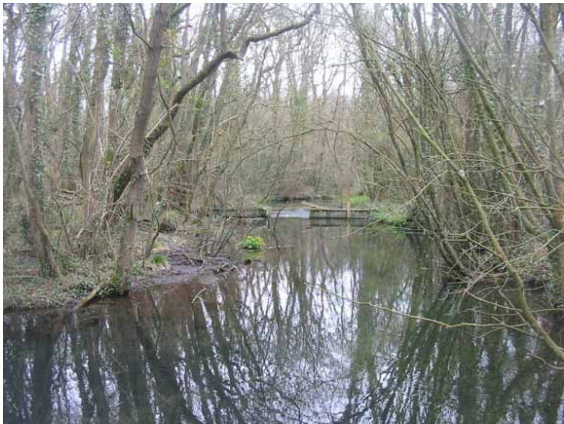
Larger impounding weir and wider, silt laden reach upstream
