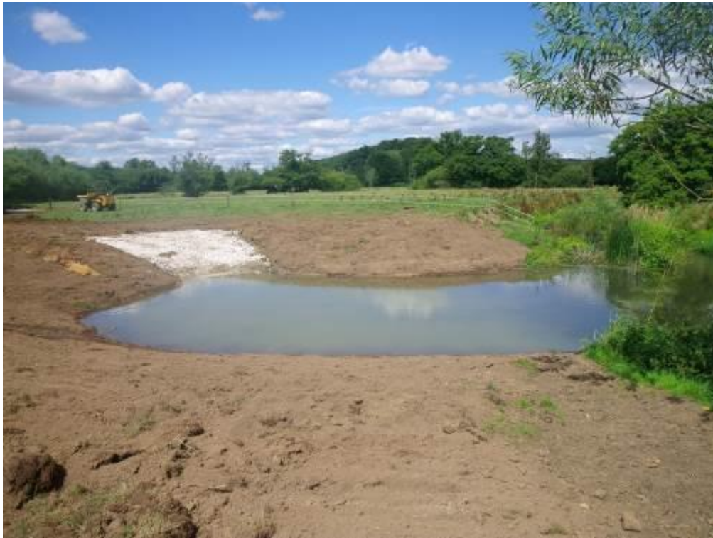
Photo 7. Recently constructed backwater on the Western Rother. When monitored, this new habitat supported seven different species of juvenile fish. The backwater doubles up as a cattle drinking bay, now fenced off from the river.
