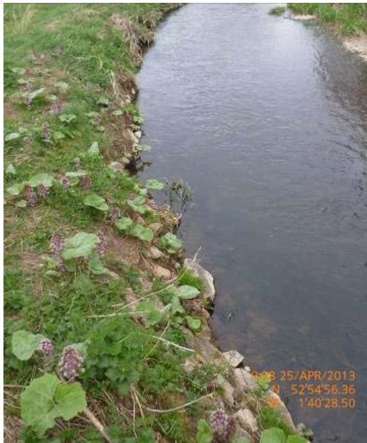
**Photo 4 Stone pitching at the toe of the bank – common to many watercourses in this area and dating back to River / Water Authority land drainage works.**
