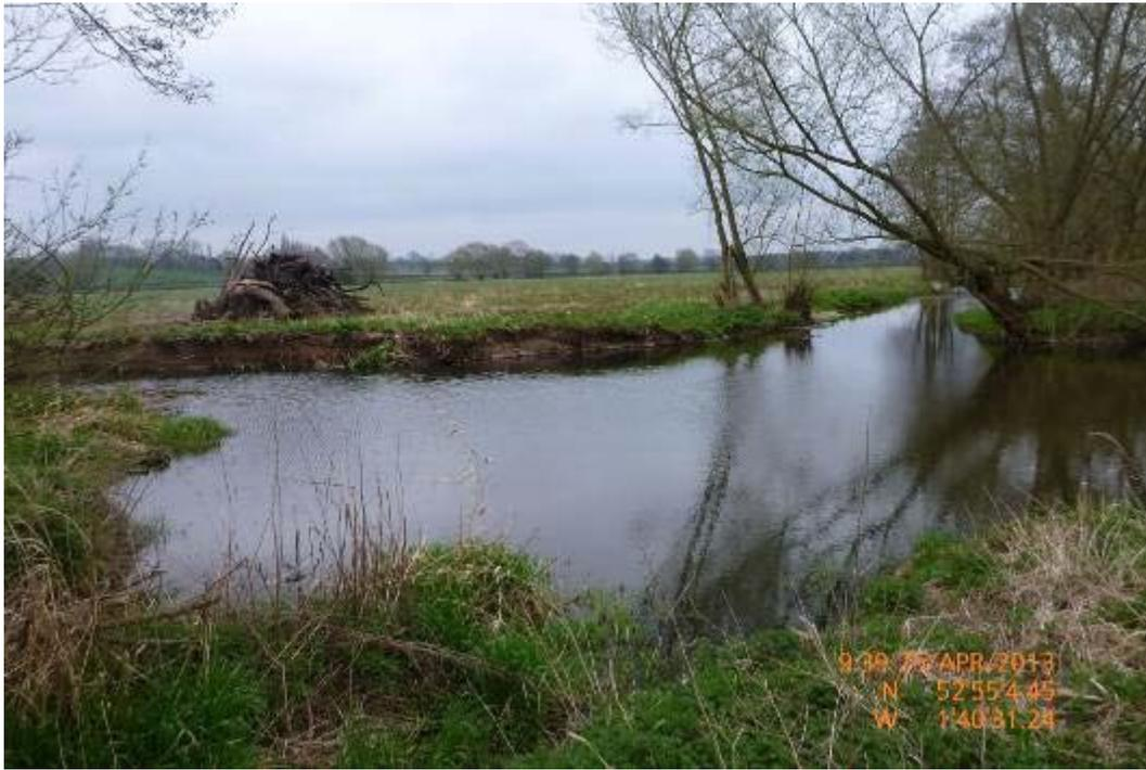
**Photo 3 More recent river engineering where the inside of a meander has been removed (far bank), further straightening and over-widening the channel to the detriment of in-stream habitat.**
