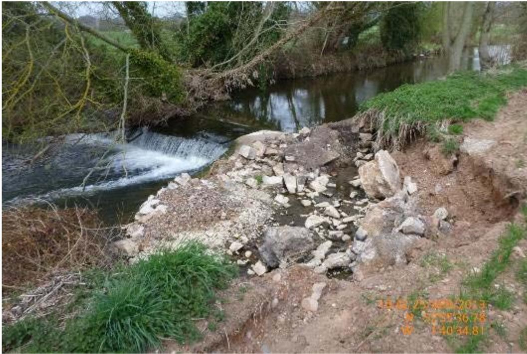
**Photo 10 Breached weir – removal of the weir is probably the best option here.**
