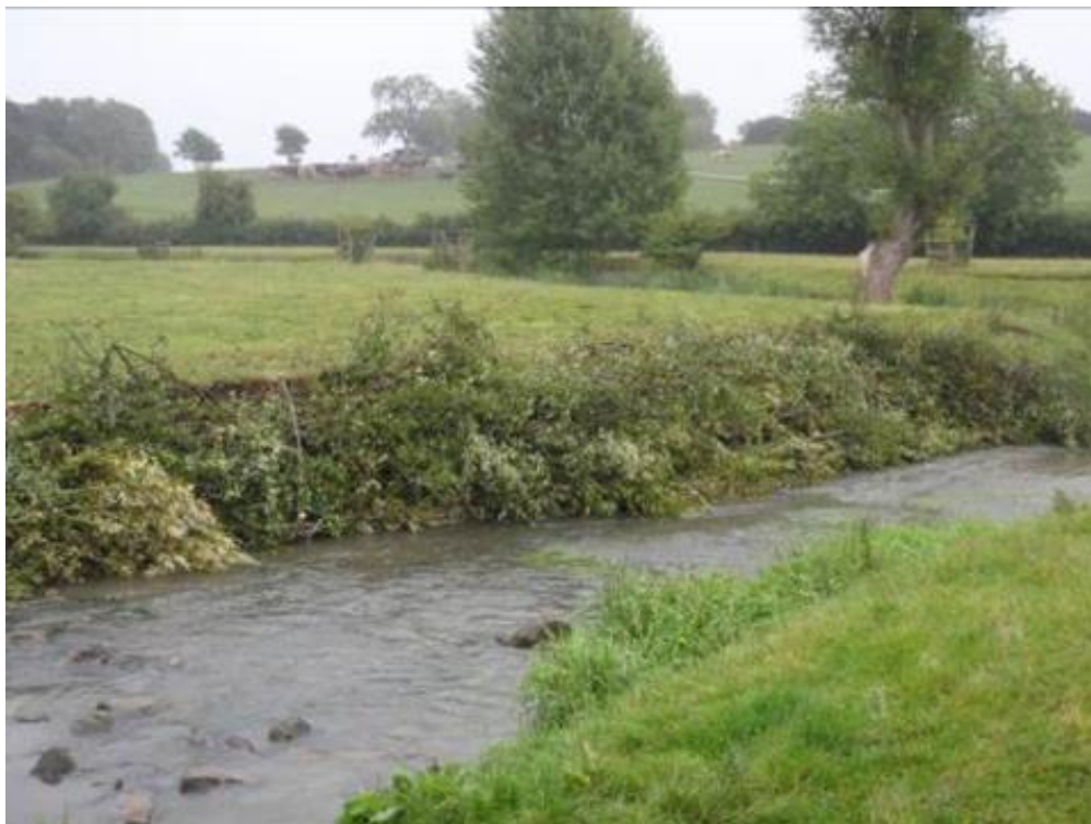
Photo 3. Depicts an eroding bank packed with brushwood.
