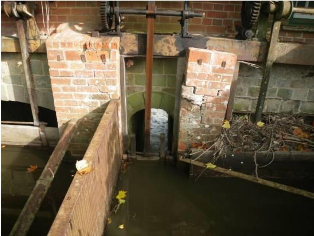
Photo 4 Eel house sluice.
