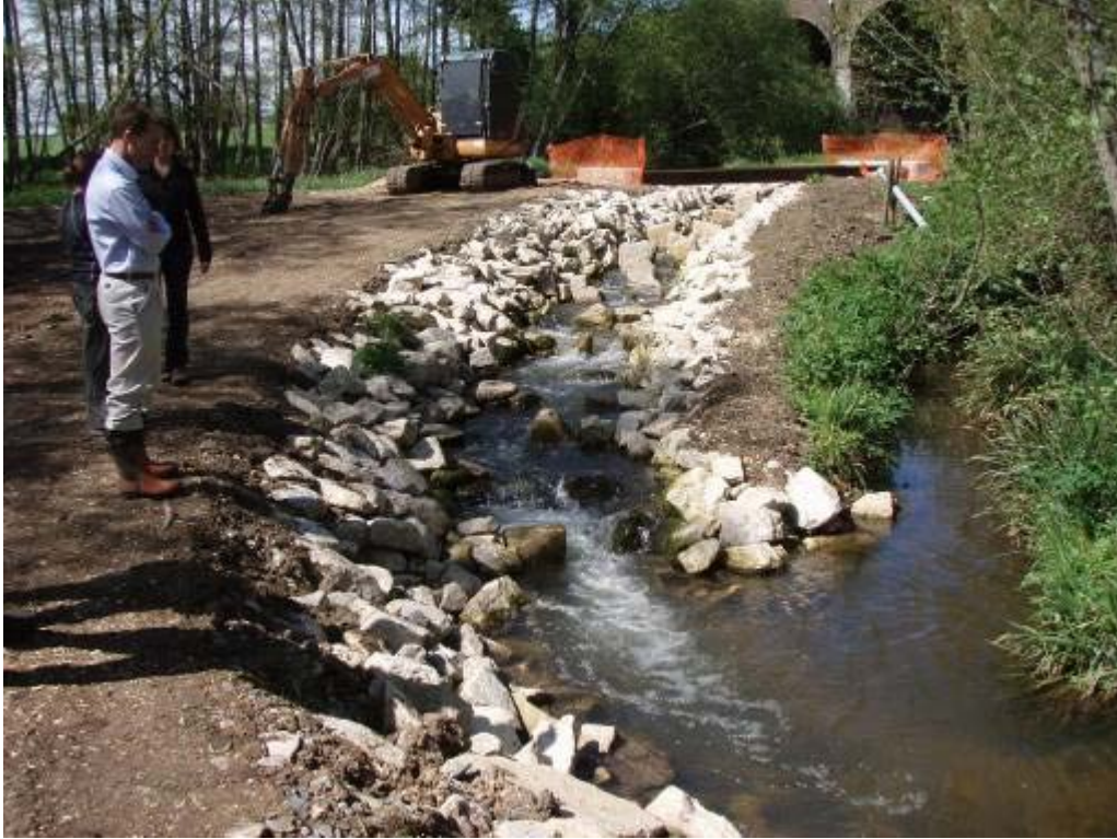
Photo 15 Nature-like fish bypass channel. A scaled-up version designed to work at different flow stages would be an improvement on existing arrangements at St. Mary's Loch outflow.
