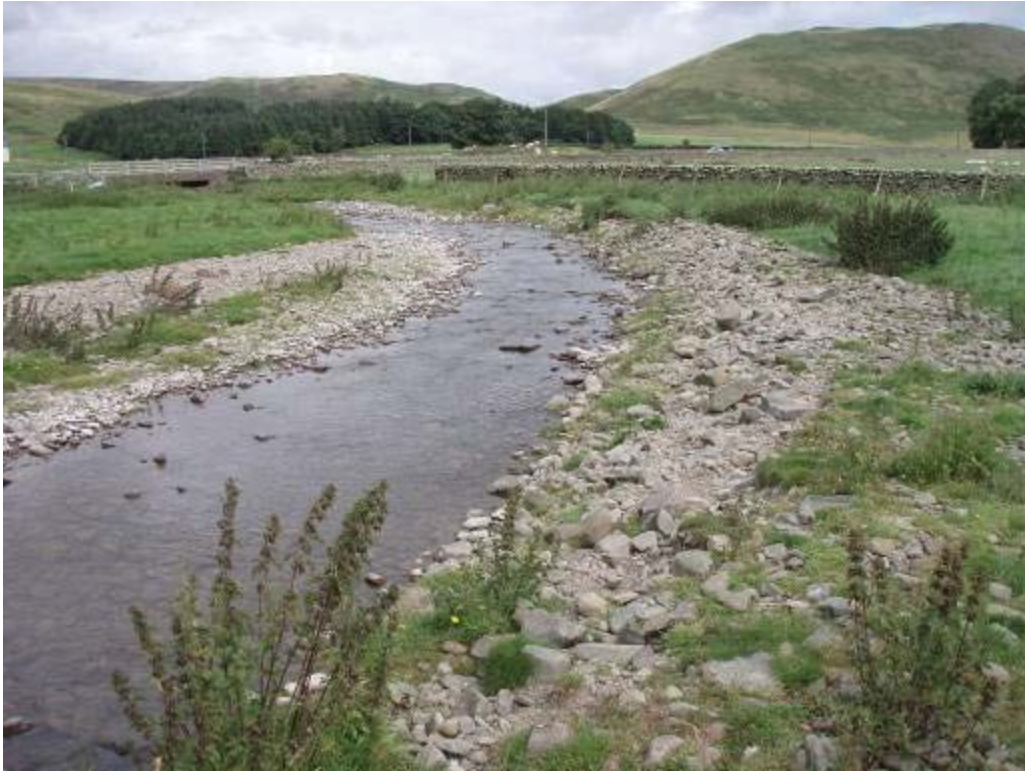
Photo 6 A little further upstream from Photo 5 (Kirkstead Burn). The channel bed has been scraped back against the outside of the bend, reducing the habitat quality of the channel still further.
