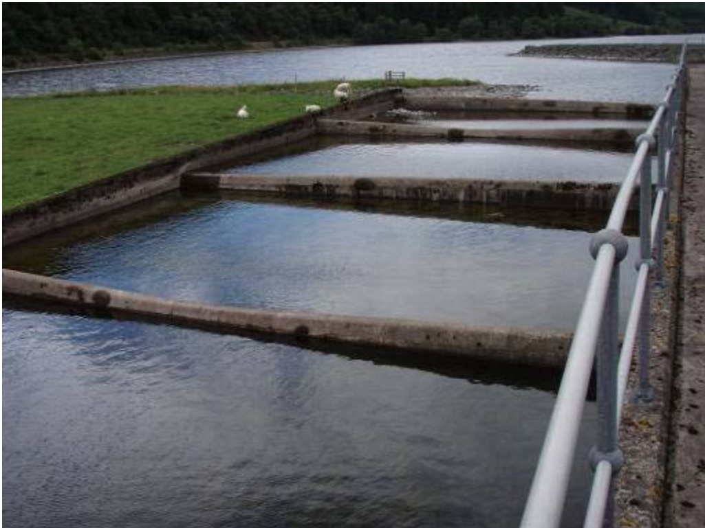
Photo 4 Channel with low weirs, not flowing at the time of the visit
