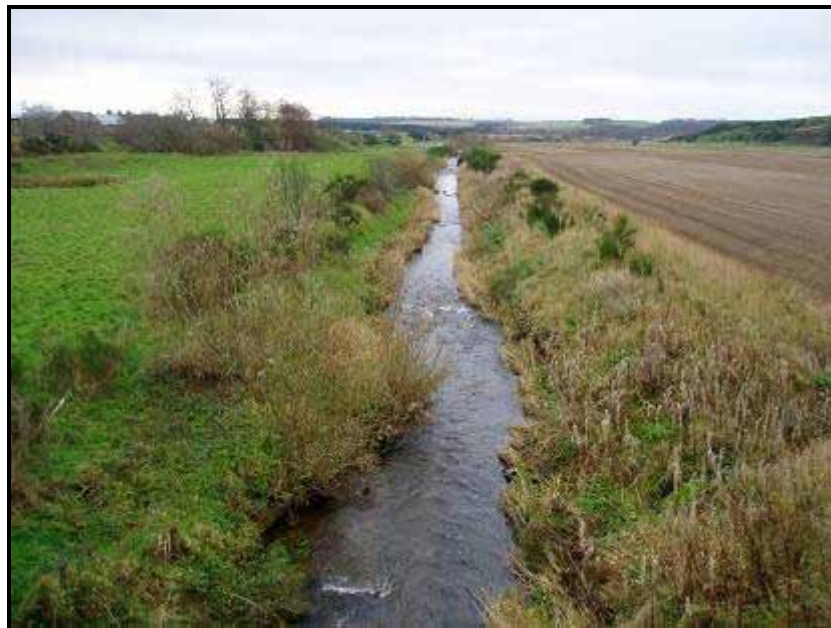
Plate XVII: Straightened burn in the River Deveron catchment showing gradual return to riffle/pool sequence
