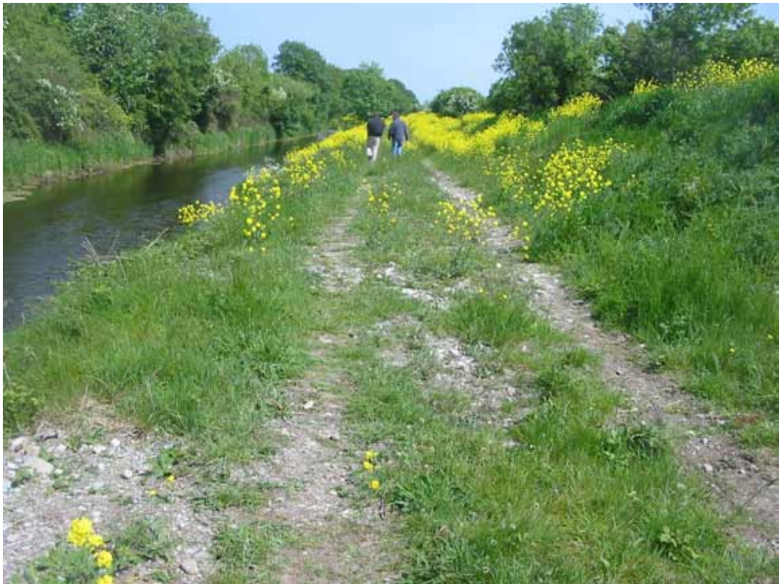
Recently excavated gravel used to make up a track on LB u/s of Iron Bridge.
