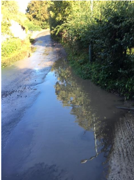
Photo 1 Massive amounts of sediment washed down the road directly into the river. (SU 31629 63648)
