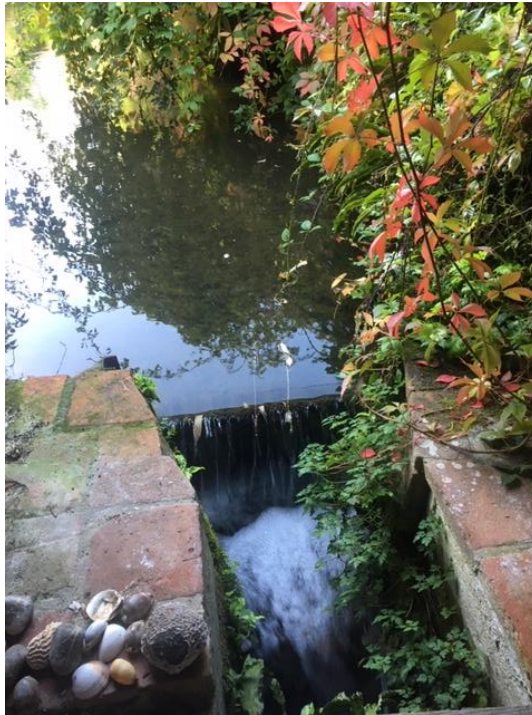
Photo 4 Boards in the old mill race, impounding the flow and impeding fish passage.
