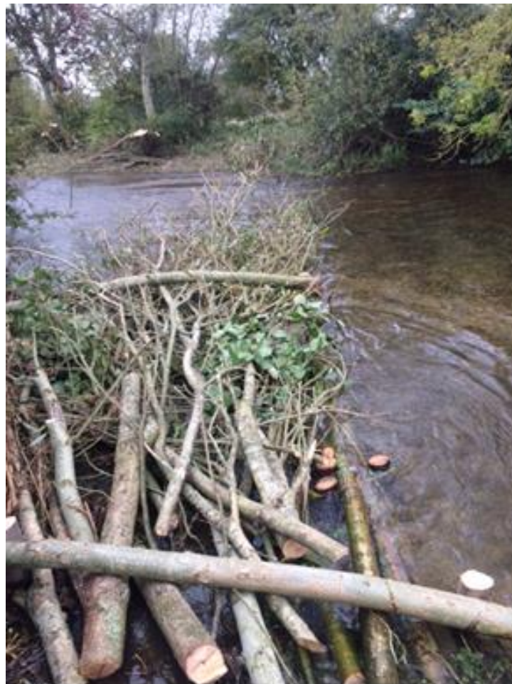
Photo 10. Brushwood mattress constructed with coppiced willow.
