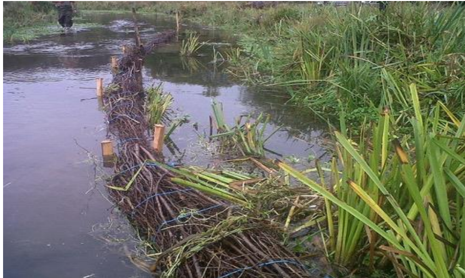
Photo 9. Faggots on the Upper Itchen used to narrow the river to help establish a margin.
