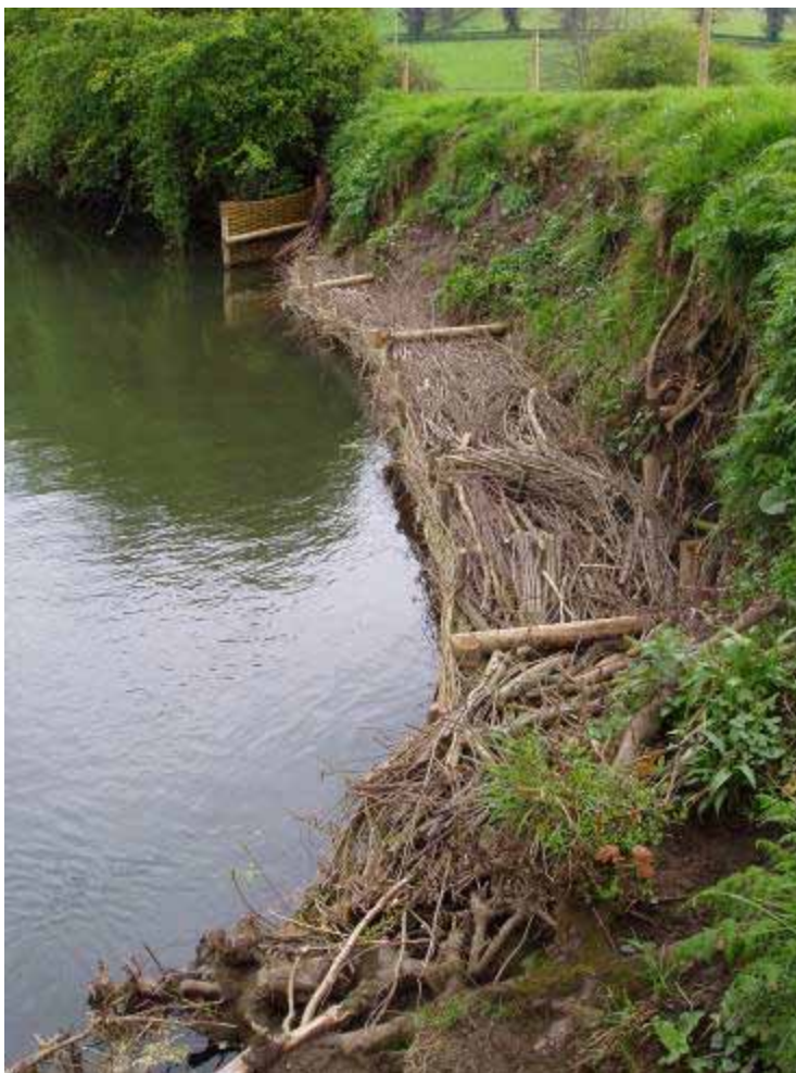
Photo 14 Brushwood protection of an eroding bank on the River Dove, Derbyshire
