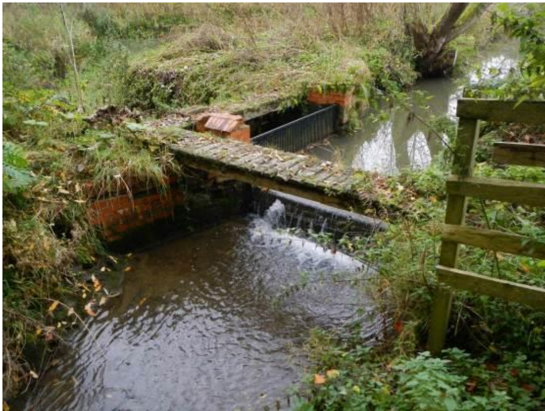
Figure 25. Weir/water feed to Settrington mill pond – a major barrier to fish passage and impoundment to beck flows.
