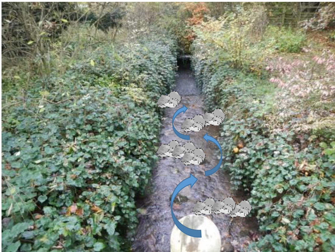
Figure 51. Boulders placed in channel to assist fish passage. The blue arrows indicate the direction of flow.
