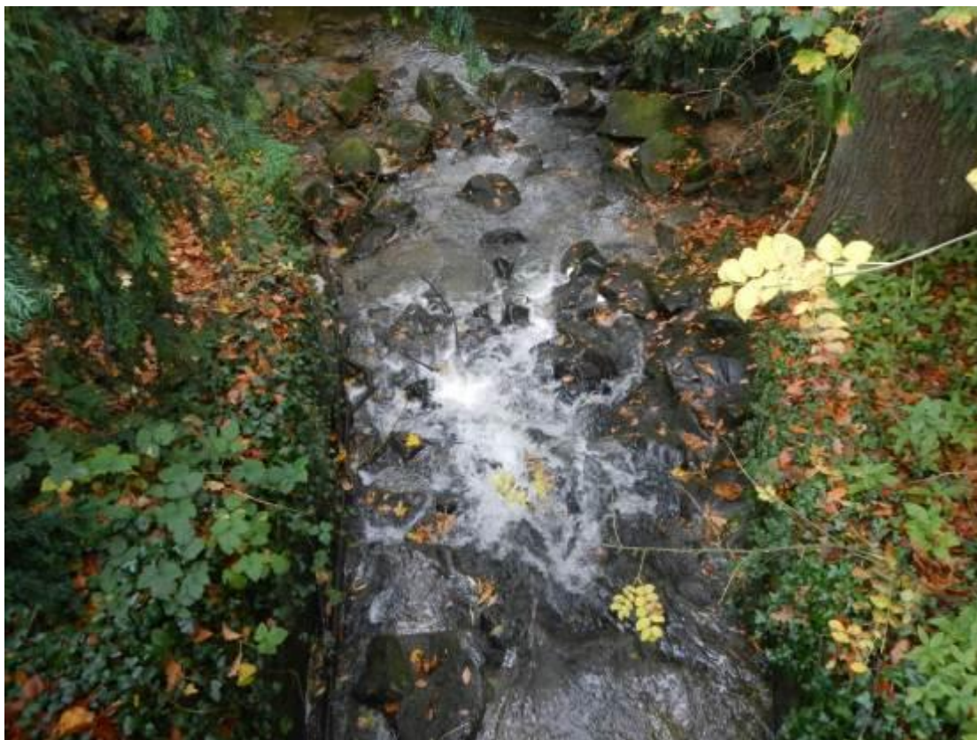
Figure 29. Rock armouring on the d/s side of the road culvert. This was likely installed as scour protection for the bed but does provide some improvement to fish passage, rather than a sheer drop or concrete lined channel.
