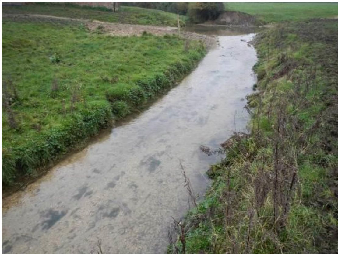
Figure 11. Straightened, over-capacity section between the two fords. Note the fine sediment composition of the substrate.
