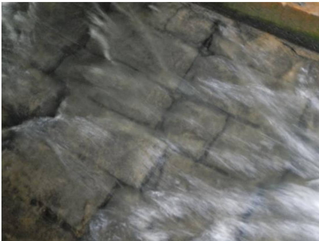
Figure 48. The swift flow over the relatively smooth and flat bed further impedes the passage of any fish making it into the culvert.
