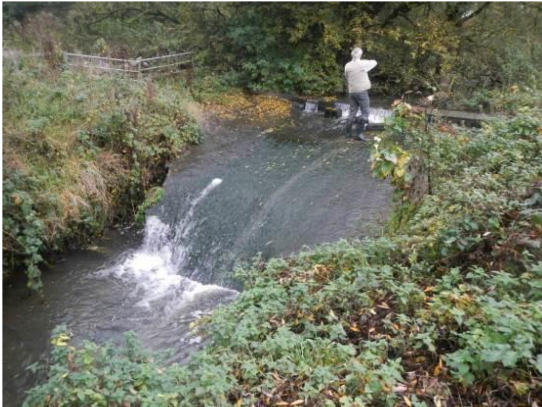
Figure 43. >3m high weir that impounds several hundred metres of the beck and poses a completely impassable barrier to the u/s migration of fish.
