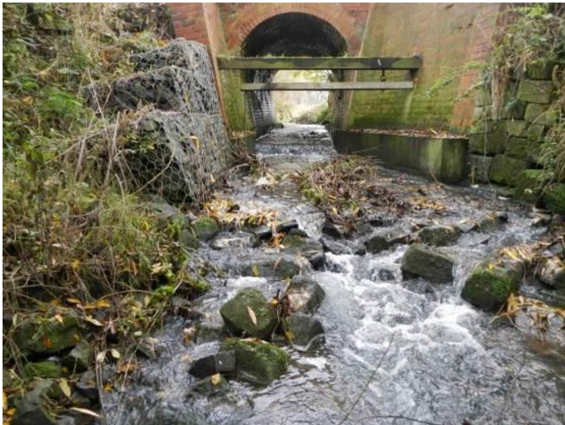
Figure 47. Railway culvert – rip rap at the d/s entrance improves fish passage somewhat, but it remains a major obstacle.
