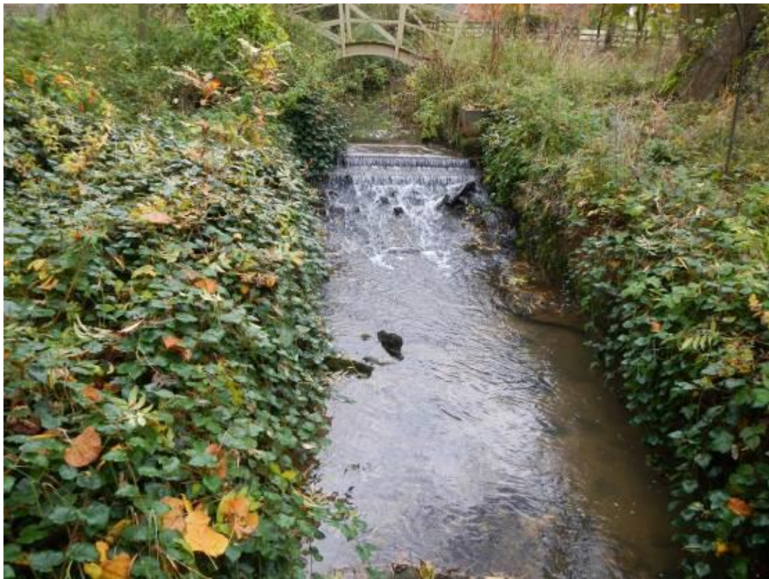
Figure 27. An ornamental weir located near the d/s end of the mill pond; an obstacle to fish passage.
