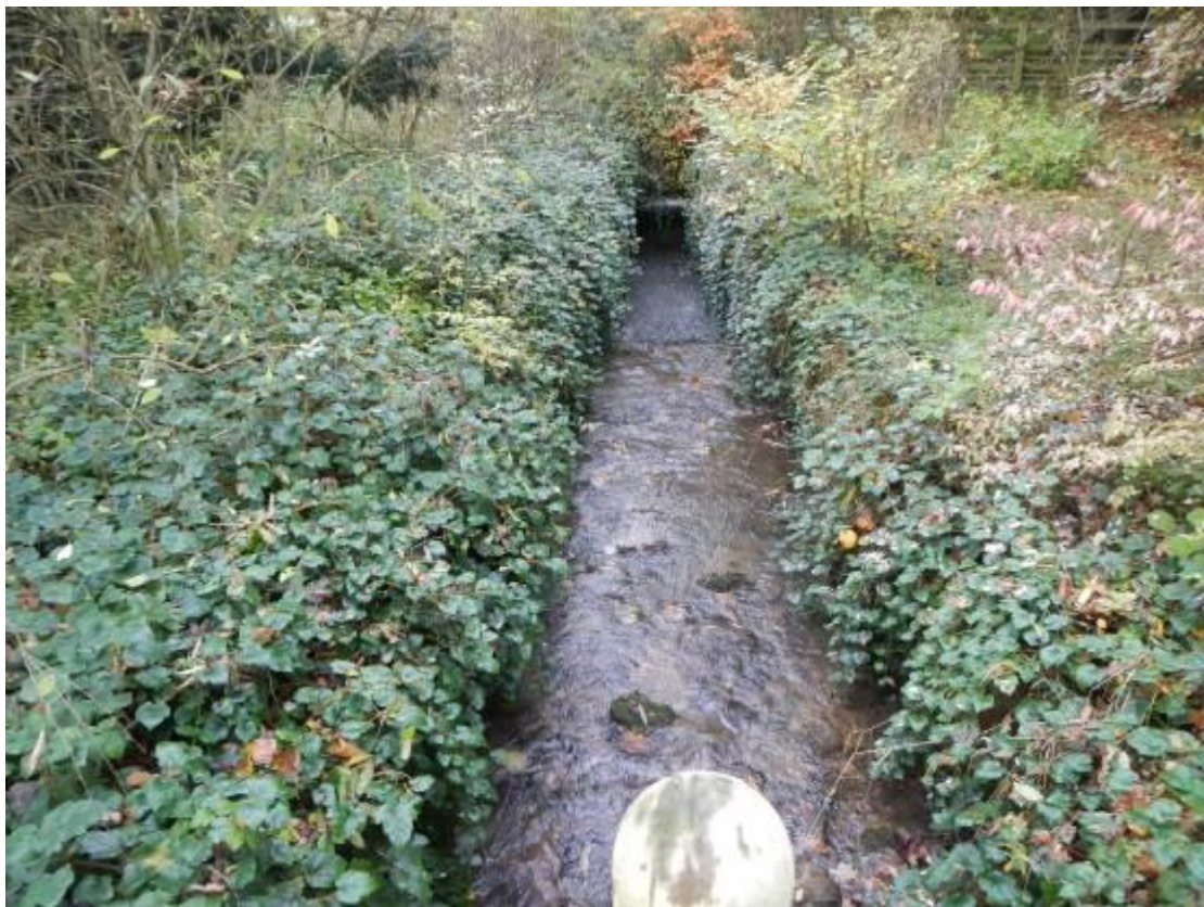
Figure 28. Poor passage for fish created by the straight, steep channel flowing down into the concrete-lined road culvert.
