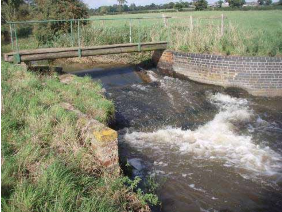
Photo 19 Weir on the Sence upstream of Bosworth Brook confluence
