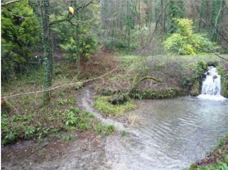
Pic 3. The large dam of the third lake has a sluice to prevent the dam from over topping. Two trout were observed getting ready to spawn on the shallow gravels in the foreground.
