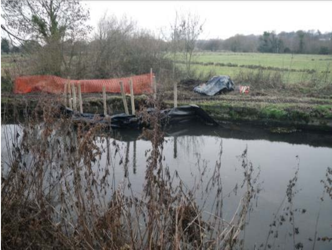
Water meadow structures under repair
