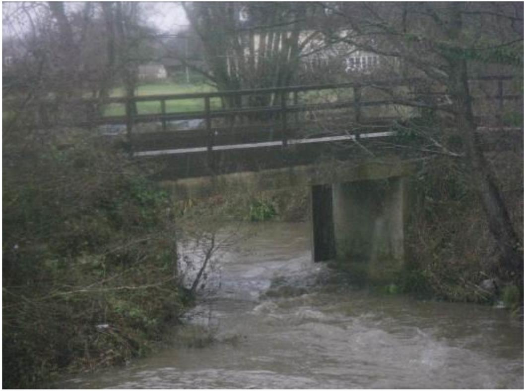
Photo 5. The high energy flume which maintains the scour pool downstream of the access bridge
