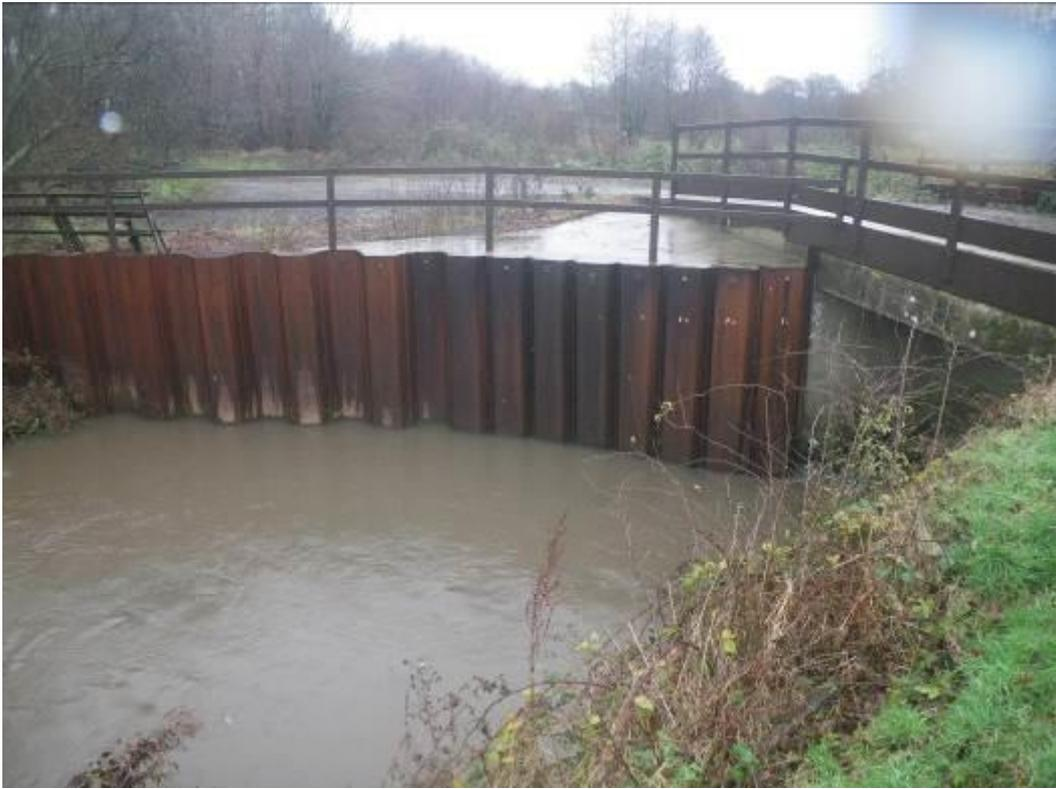
Photo 4. Installing new natural toe to the bank in front of the existing piling will help to offset the negative impacts of vertical steel piling.
