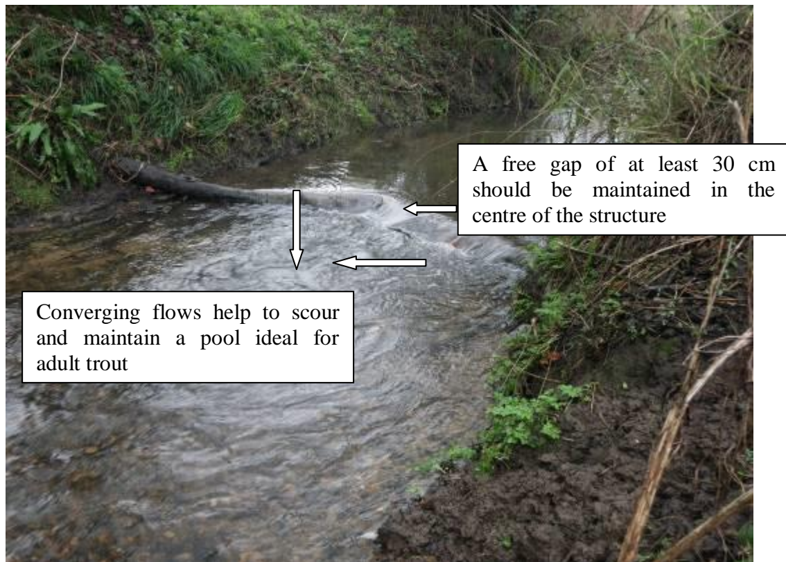
Photo 2. Upstream facing V deflectors. These can be made from tree trunks or stones.
