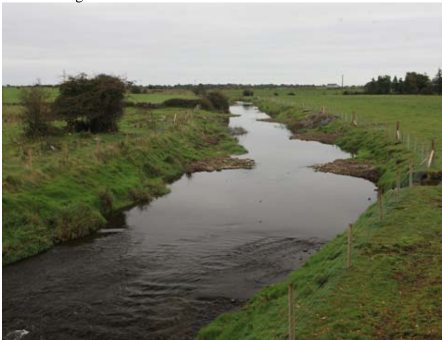
Alternating and paired deflectors installed IFI with downstream rock ramp
