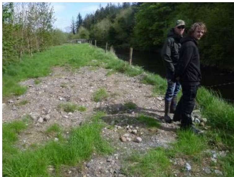
Fig 1: RRAC members standing on pile of gravel recently dredged from the river
