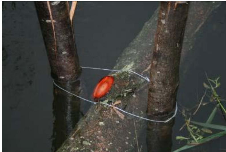
.... And additional fixing using stakes and wire
