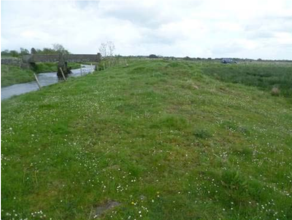
Fig. 4 Temporary fencing close to the bank top. Note also the raised bank of dredged spoil on the LB
