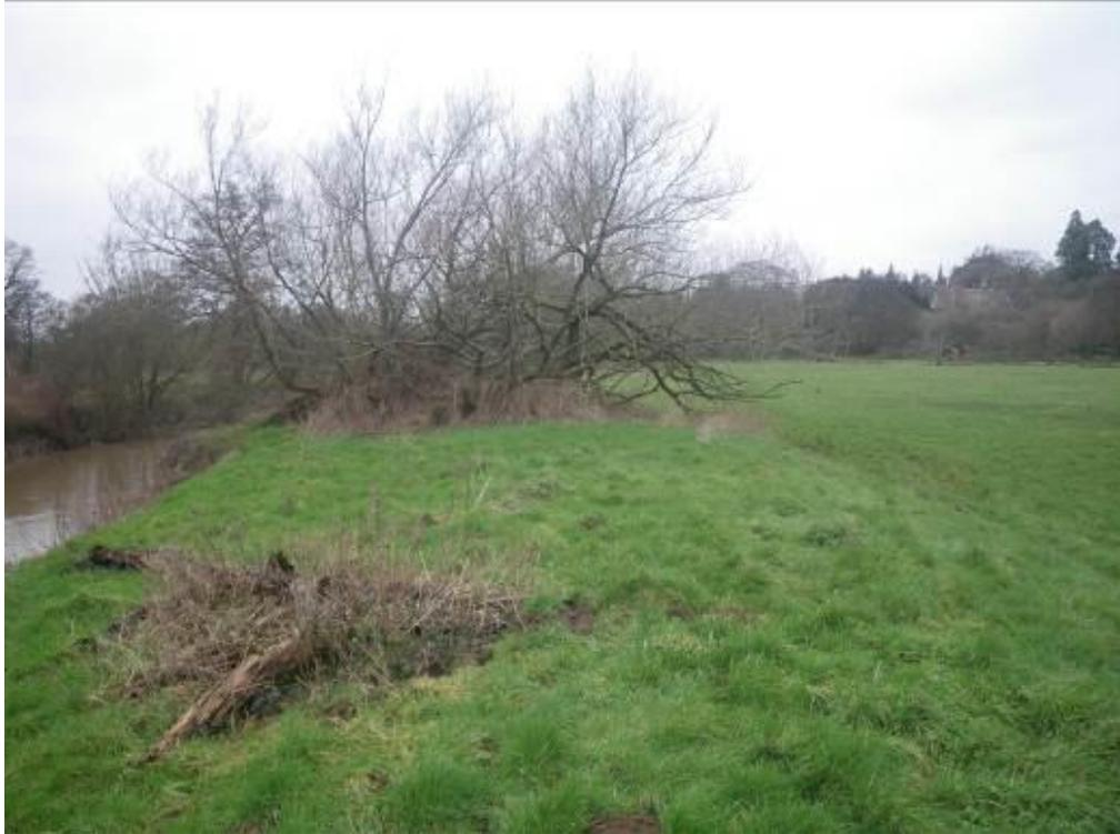
Photo 6. Where the top of the bank is raised above the adjacent flood plain. Cutting a wide notch in the bund would improve flood plain connectivity
