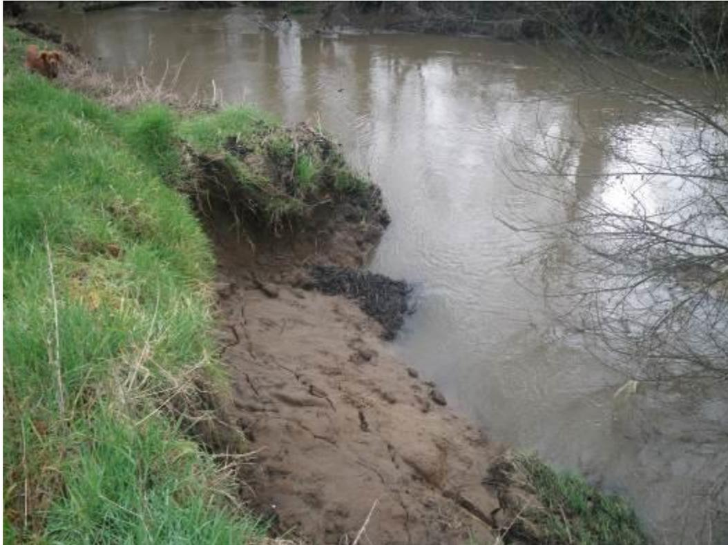
Photo 10. A section of typical Rother bank failure, in this case caused by a fallen tree opposite. These low, exposed areas can be stabilised with rooted plants to form a low, natural margin rather than a sandy cliff.
