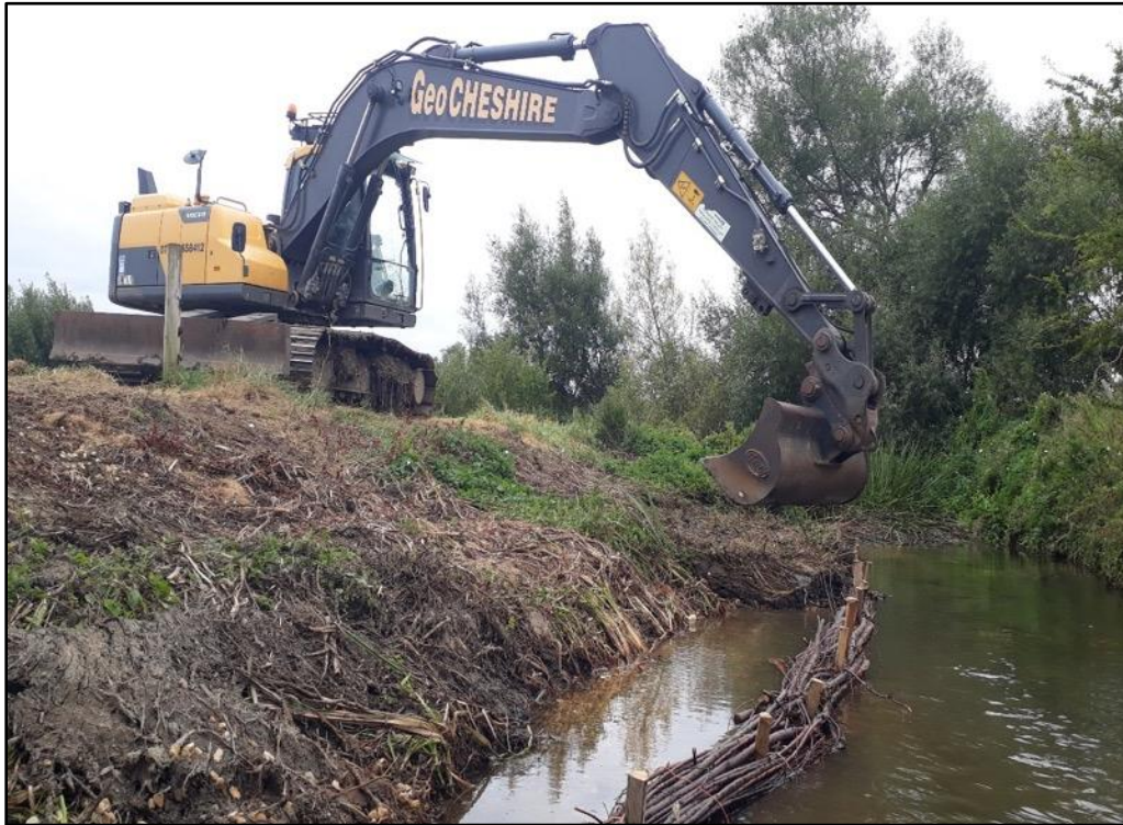
Pic 28 – An excavator can be used to re-grade banks, pushing existing material down and out into the channel.
