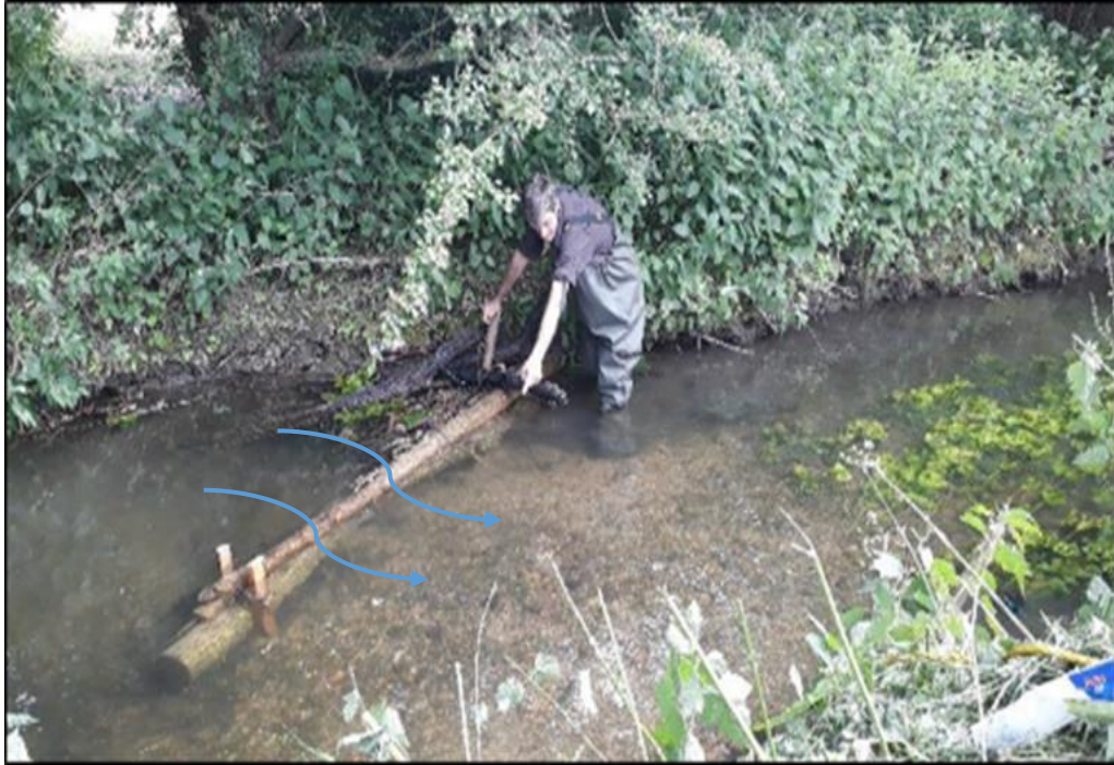
Pic 26 - A flow deflector used to focus flow and scour into the centre of a river.
