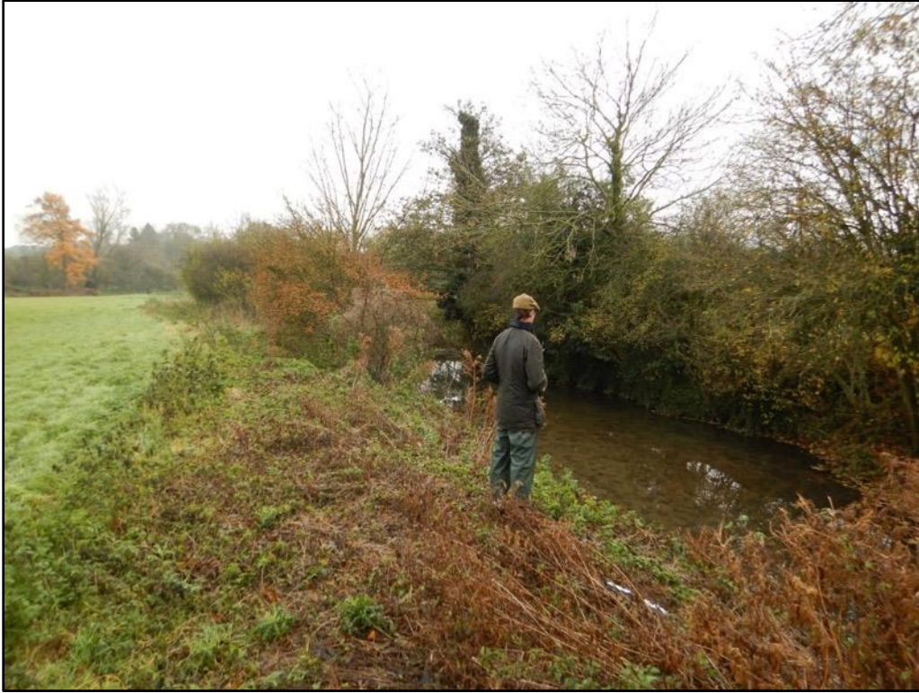
Pic 18 (TL 39207 23771) – This length of bank could be pushed down and into the river, to create a narrowed low-flow river with a 2-stage channel.
