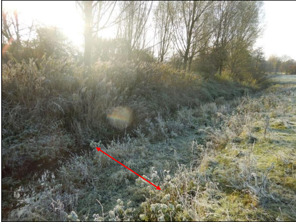
Pic 6 (TL 39138 24229) – The river has narrowed to create a significant vegetated berm (red arrow) resulting in the 2-stage channel.
