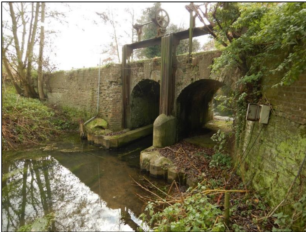
Pic 13 (TL 39123 23884) – The bridge footings and historic sluice arrangement no longer present a barrier to fish movement.
