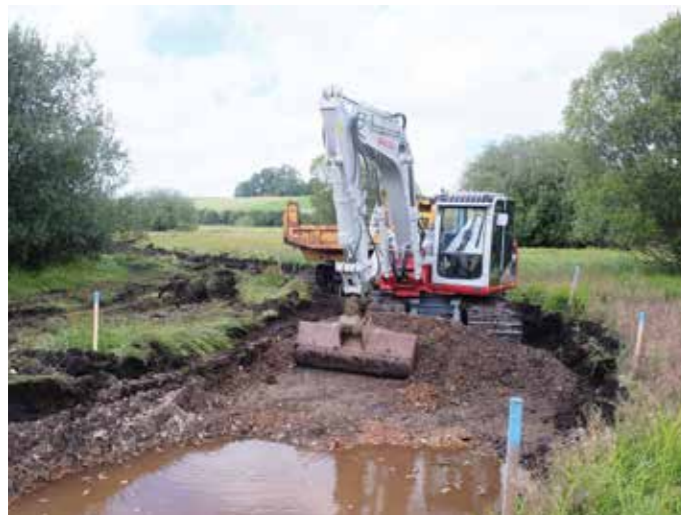
Pre works: Using a digger to re-create the natural channel
