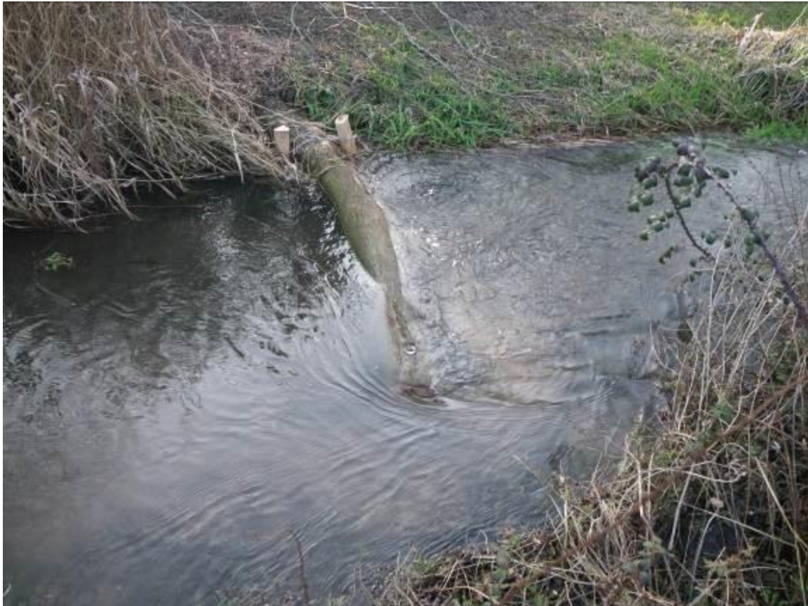
Photo 9. Typical tree trunk deflector designed to create local bed scour and sorting of bed sediments. This stream is flowing from left to right of shot.
