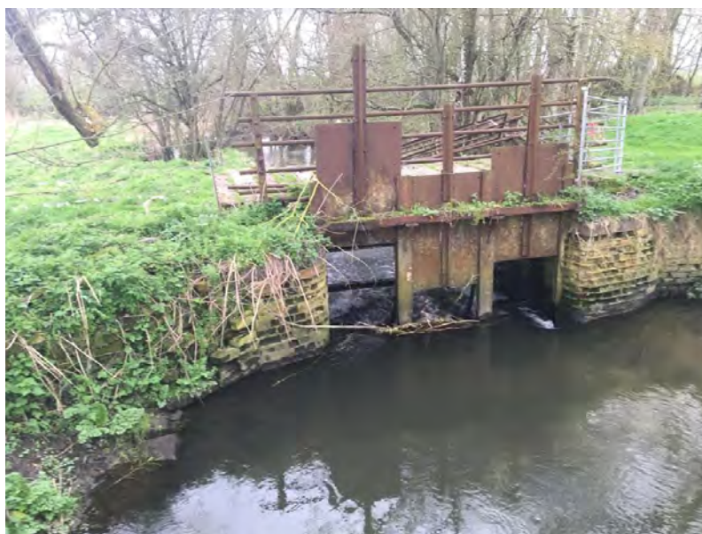
Photo 10. Old derelict hatches, previously used to flood the watermeadow being reconnected in the project by the WWT.
