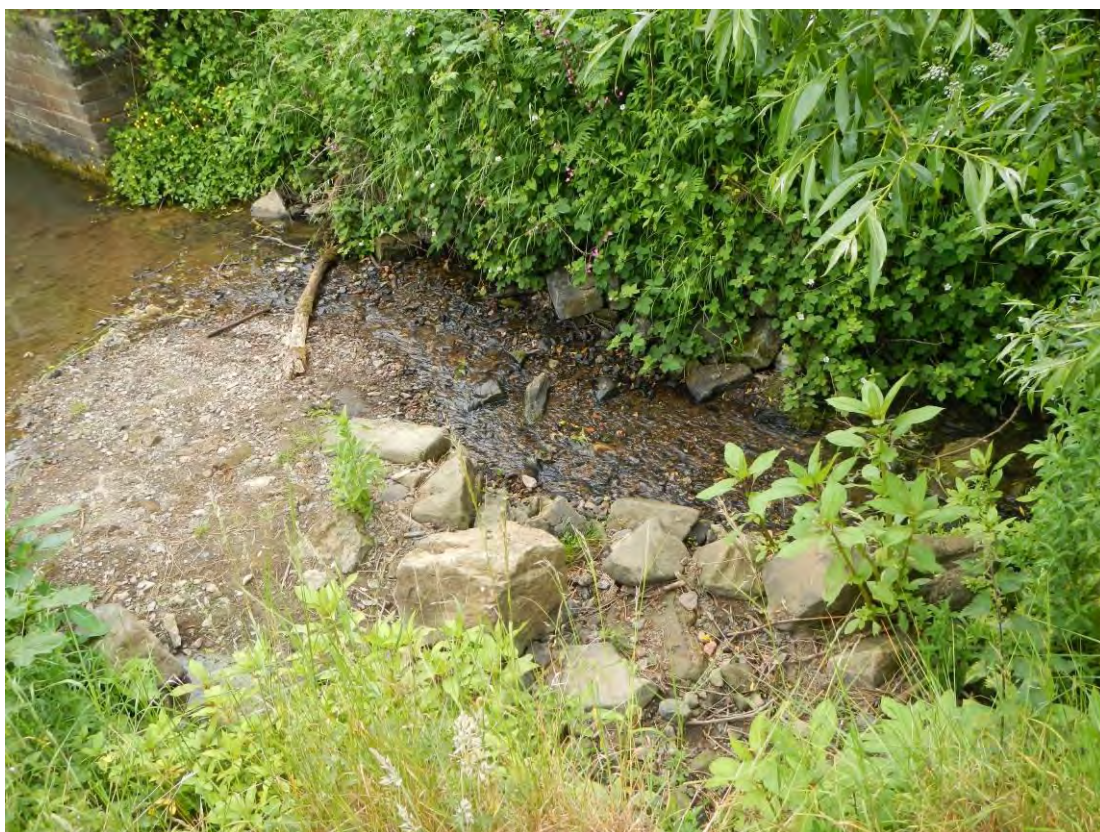
Figure 20. Bank erosion on tributary, just d/s of culvert. The issue is greatly exacerbated by Himalayan balsam and unsympathetic rock armouring. Creating a naturally vegetated, more stable bank and therefore appropriate channel width to develop should assist with sorting of the substrate.
