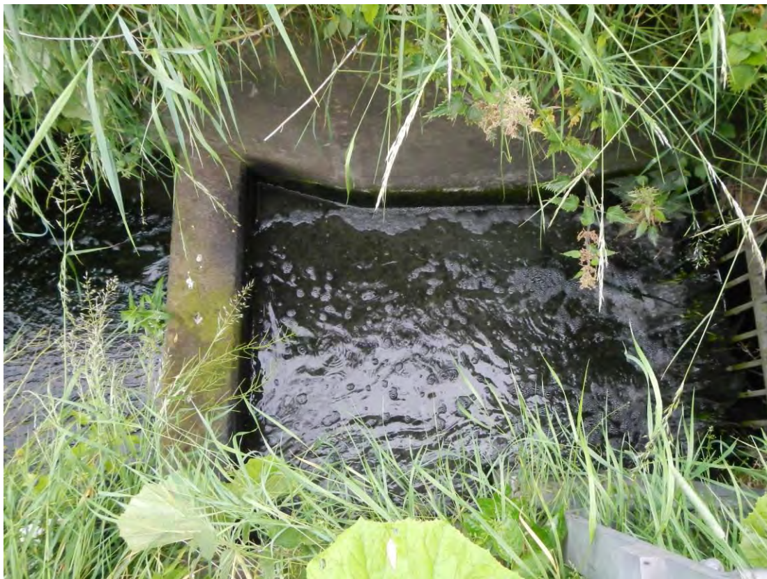
Figure 13. The STW outfall. Note the grey coating on the bed of the channel. This indicates high nutrient/poorly treated water emanates from the outfall at times – something that should be closely monitored, and reported when observed.
