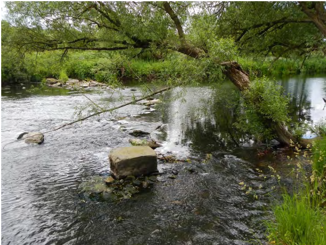
Figure 18. Bank erosion issues where another stone weir has been out-flanked by flows.
