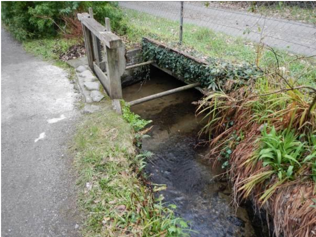
Figure 19. Sluice that further splits flow from the main flow of the tributary and supplies the small channel re-joining the main channel d/s of the falls in section depicted in Figure 21.
