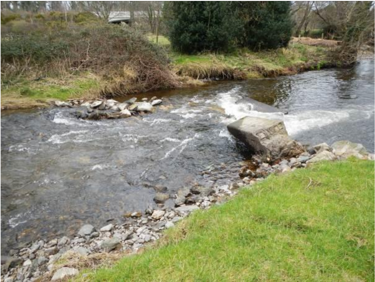
Figure 30. Collapsed d/s paired deflector that would have focussed flows to the centre of the channel at low water but deflected any high flows that overtopped the structure into the banks, causing erosion and widening the channel.
