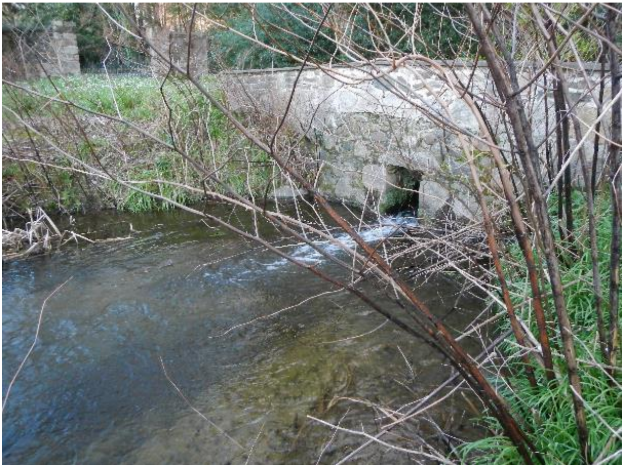
Figure 18. Sluice feeding a pond and additional channel d/s of the pond from the main tributary. In addition to poor passability through the sluice, an overspill at the d/s end of the pond also restricts u/s migration via this route. Also note the Japanese knotweed (brown canes - right of shot).
