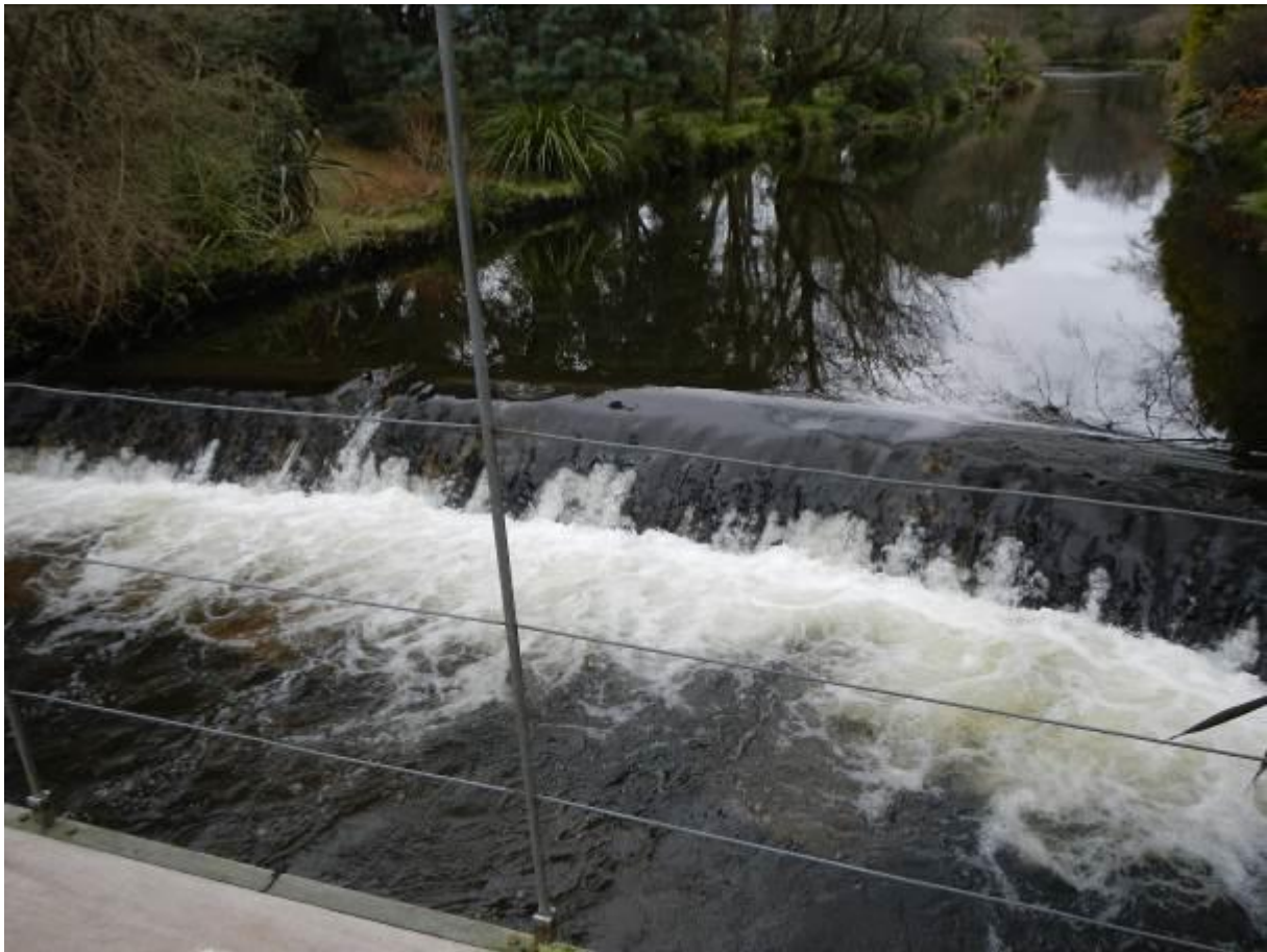
Figure 13. The largest weir in Mt. Usher Gardens. This is a sizeable obstruction and likely to inhibit fish passage, particularly at low flows and for the vital smaller/juvenile fish that are often overlooked.
