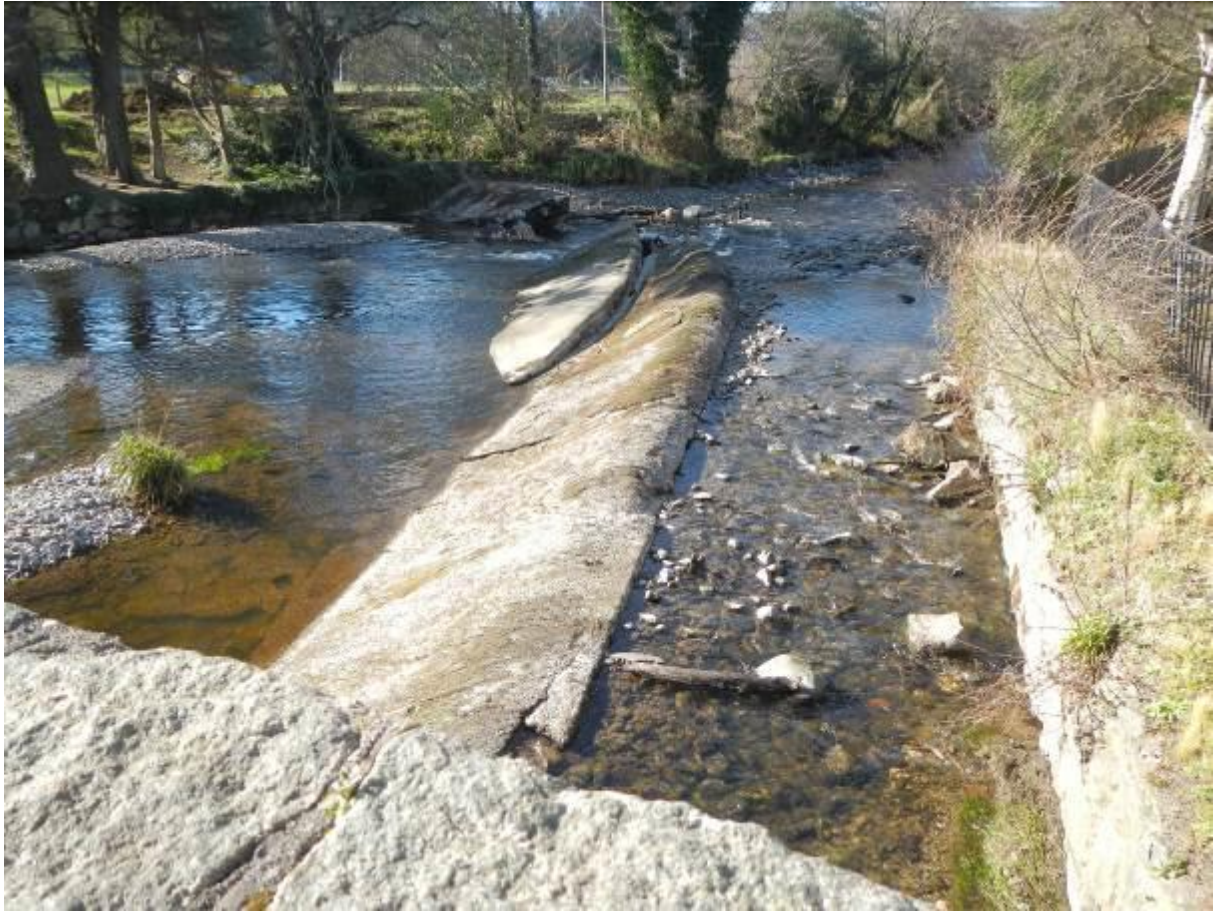
Figure 10. The remains of Ashford Weir. Collapse of the central section of this weir has facilitated the significant habitat improvements u/s, reinstated sediment transport through the area and greatly improved habitat connectivity/fish passage.
