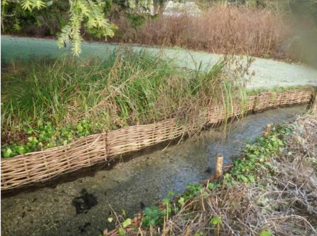
Photo 2 Hazel hurdle revetment on the by-wash channel.
