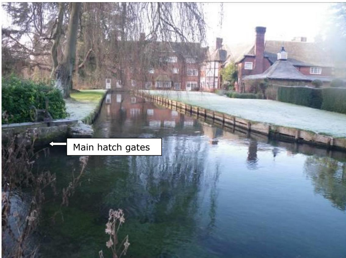
Photo 3. Main river hatches used to regulate upstream water levels and flow splits between the channels
