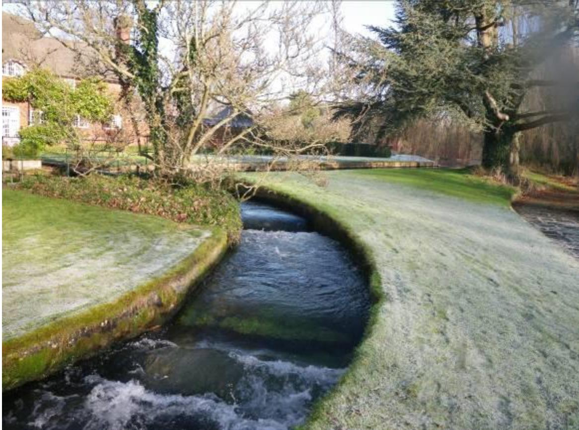
Photo 4. The 'fish pass' pool and traverse sequence which bypasses the mill wheel and provides a usable safe route for upstream migration. Maintaining strong flows via this route will be very important in the autumn/early winter period.
