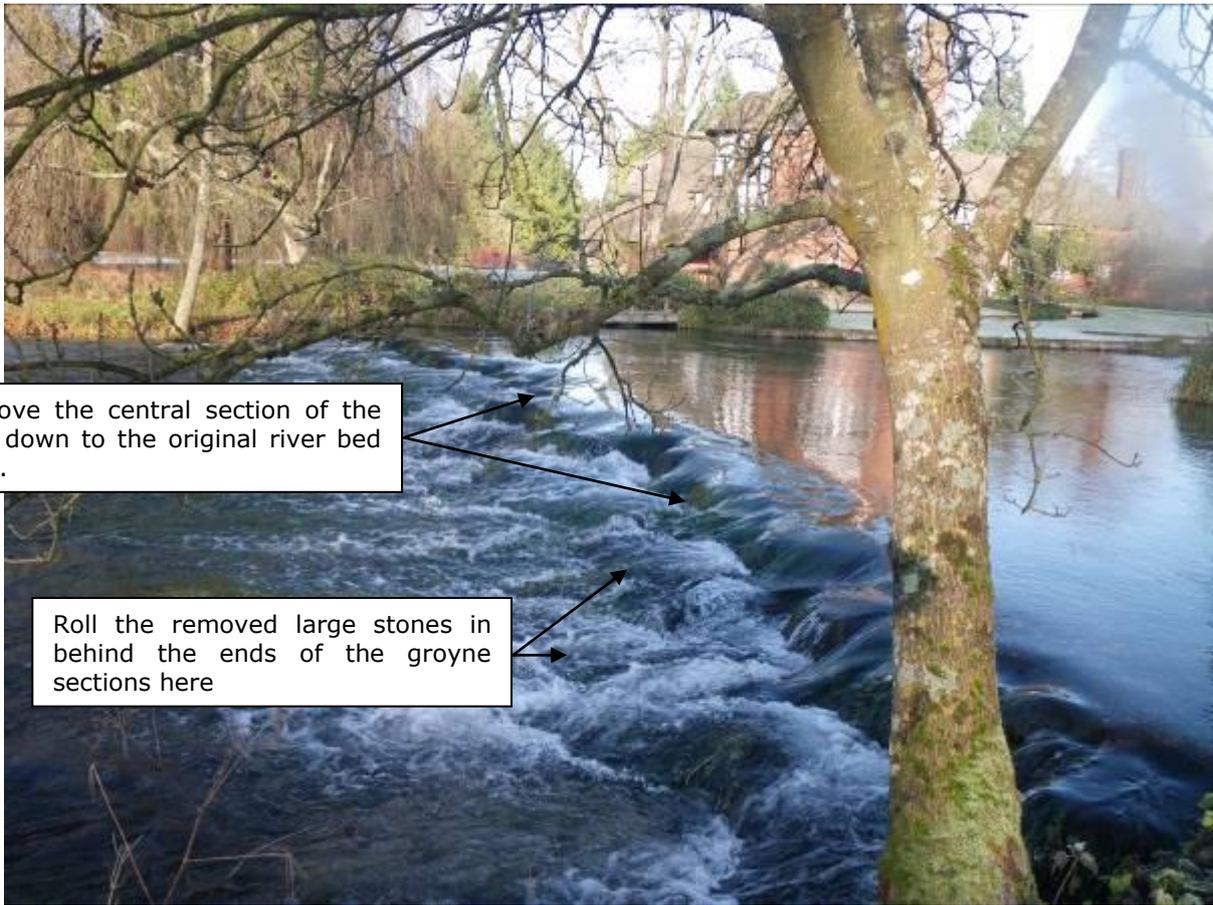
Photo 5. The blockstone adjacent to the house could be modified to improve in-channel habitat
