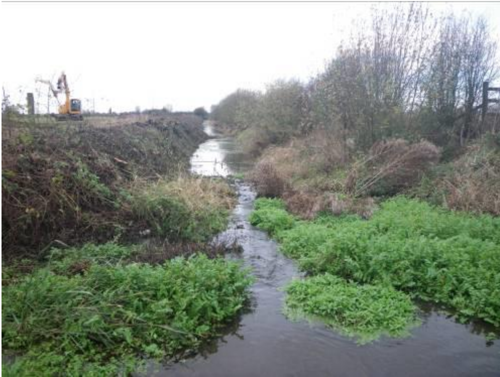
Photo 3. Looking downstream of the ford at the straightened channel
