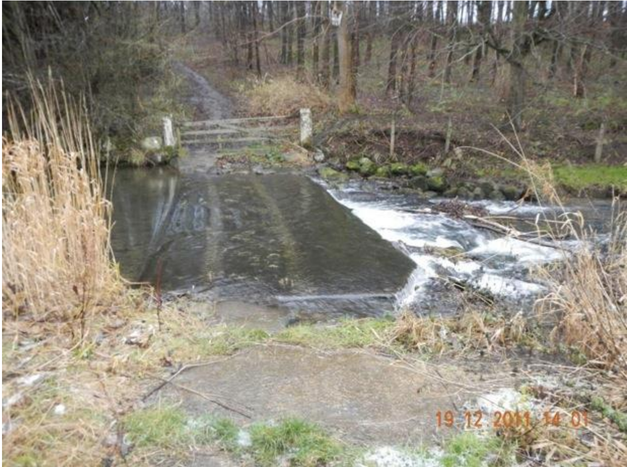
Picture 13. Concrete ford which poses a barrier to juvenile fish migration, and adult fish migration at low flows (NZ1148571797).
