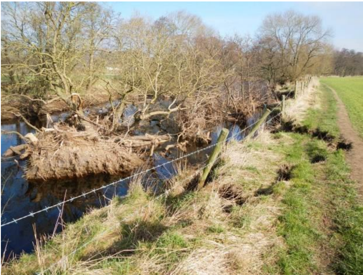
Figure 3. Large accumulation of trees/woody material and bank erosion, immediately d/s of sheet piling in the bank which has undoubtedly deflected a greater energy of scour onto the bank in the erosion area.
