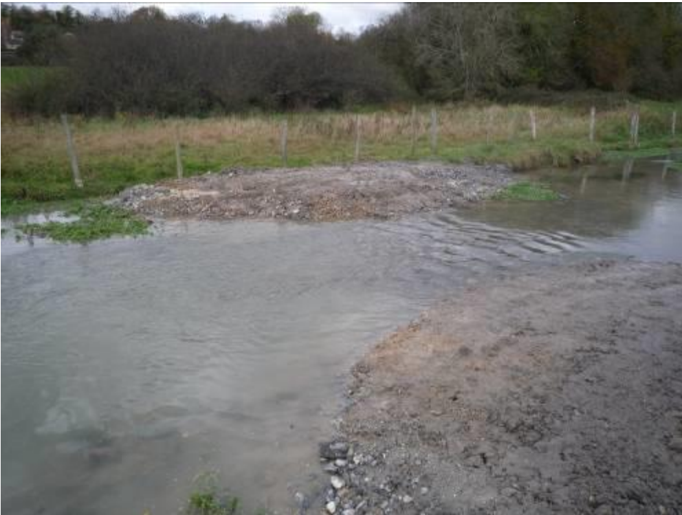
Photo 4 & 5. The “dig and dump” technique used on the River Meon in Hampshire to create a “run and a pool”
