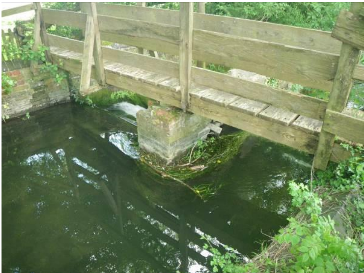
Photo 1. Access footbridge spanning double weir hatches
