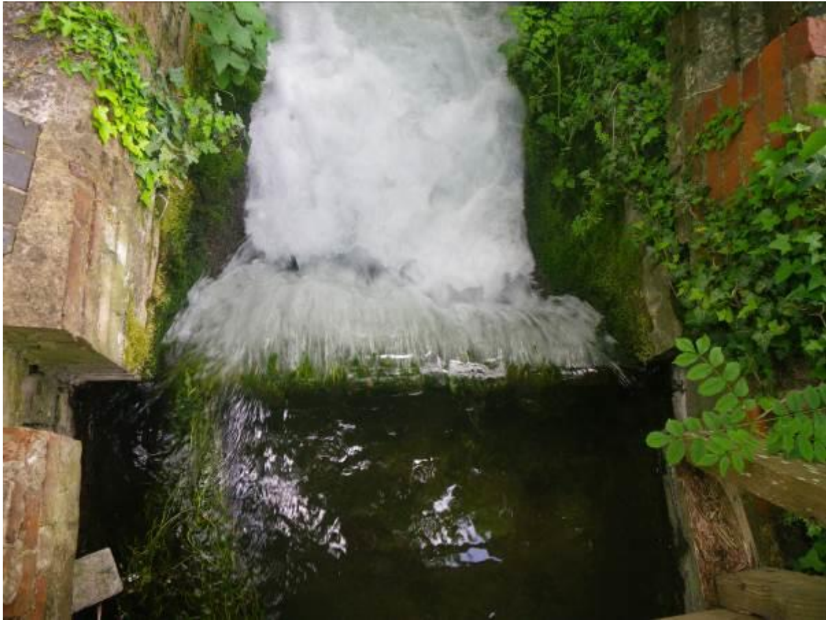
Photo 2. Significant head loss in excess of 300mm represents a blockage for all but the largest trout during high water conditions.
