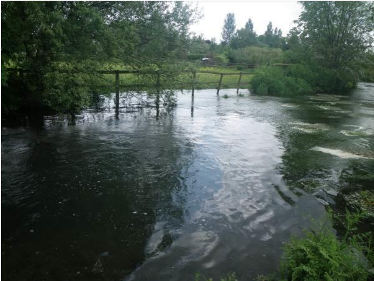
Photo 6. A drink bay adjacent to the LB needs to be managed and maintained to avoid excessive bank damage and over-widening of the channel.
