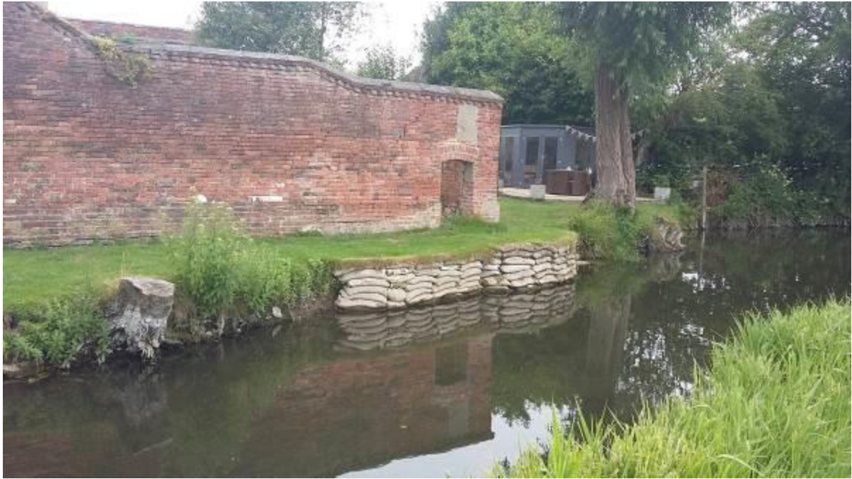
Photo 2. Highlighting the area of vulnerable bank immediately downstream of the bagwork.
