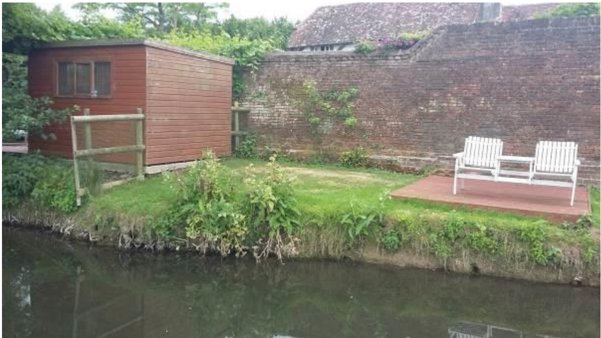
Photo 3. The vertical nature of the bank leaves it more susceptible to failure. Planting up a low, energy absorbing toe to the existing bank would create effective and attractive bank defences.
