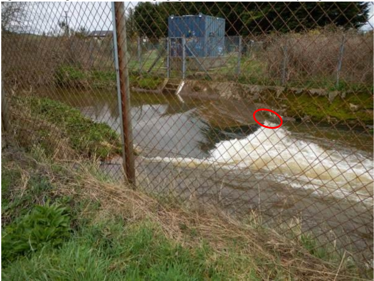
Figure 16. Side view of the flat-V gauging weir, where shallow, high velocity flows provide a physical and behavioural barrier to fish passage. Increased flow and depth that would ordinarily make an area more passable are likely to significantly inhibit fish passage through greatly increased flow velocities. The small trout was observed failing to ascend the weir in the area highlighted in red – it is probable that this was the only area with low enough velocities for the fish to even attempt the ascent.
