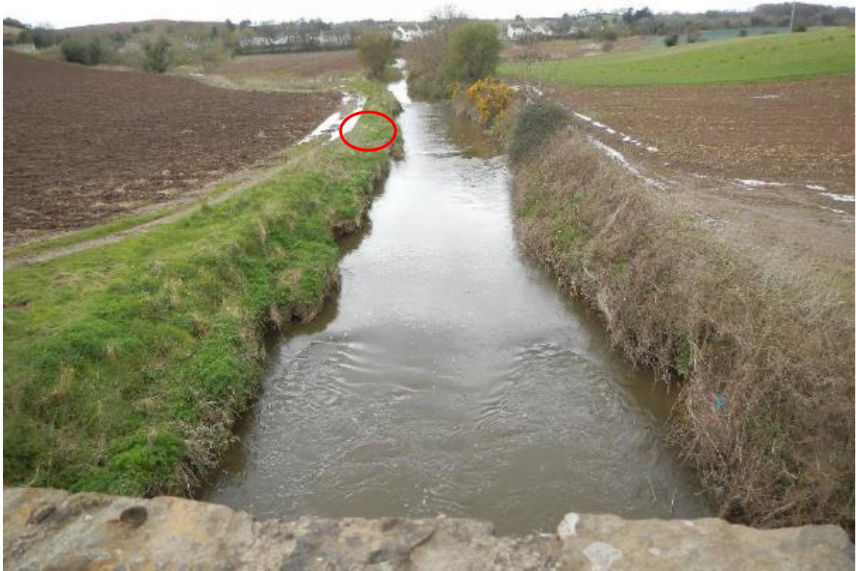
Figure 18. Looking u/s of Kennel Bridge, the channel is significantly straightened and uniform offering little refuge from predators. Drainage points from low-lying areas of track and puddles drain silt laden water directly to the river (red circle).
