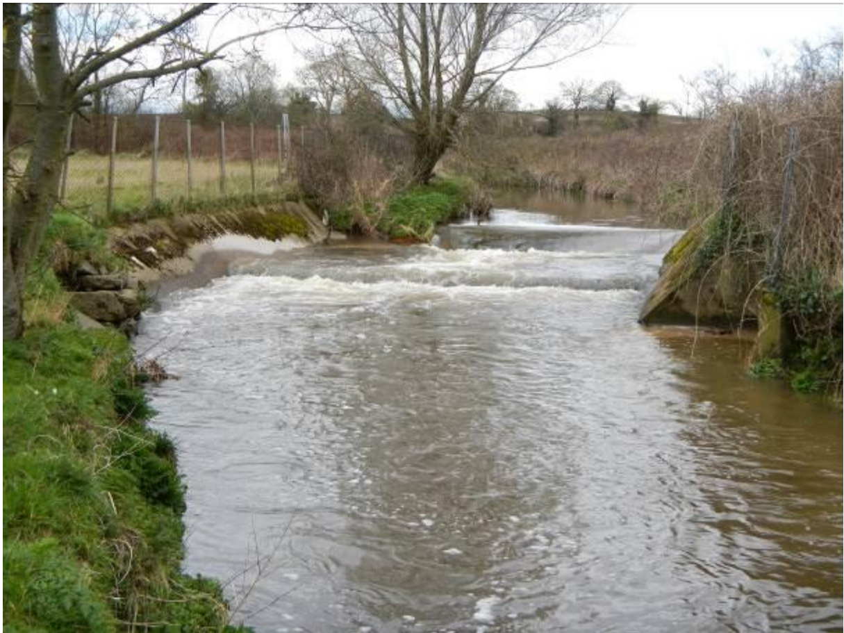
Figure 15. Looking u/s at the flat-V flow gauging weir – a notable barrier to fish passage.
