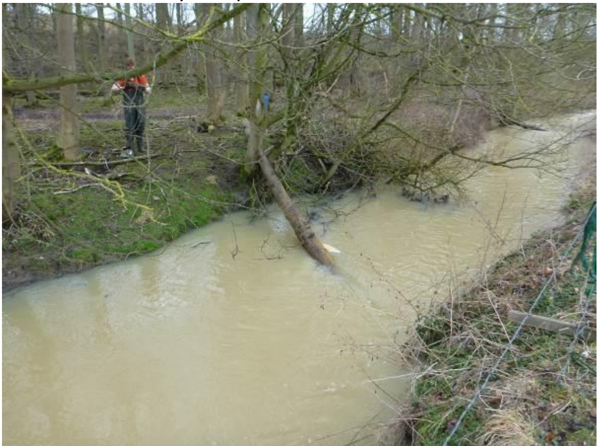
Figure 33. An alternative way of anchoring a tree kicker or log/woody material without manmade fixings. This technique simply relies on winching the butt end of the wood between two adjacent trees/branches and allowing friction to hold the material in place. Best for low flood risk areas but still a very secure method of fixing.
