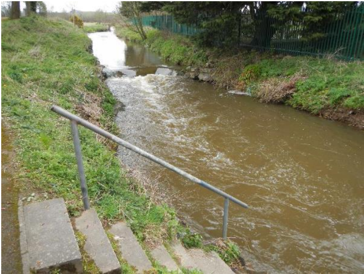
Figure 14. Another of the numerous rock weirs throughout the Middle Section that pose issues to fish and substrate movement.
