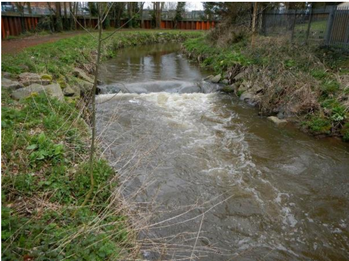
Figure 13. A potential barrier to fish movement which impounds the river u/s and interrupts sediment transport through the river.
