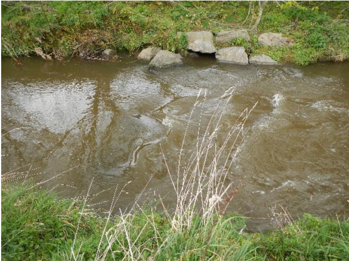
Figure 20. One of many low-level weirs in the Upper Section that impound the river and inhibit the development of a more natural channel.
