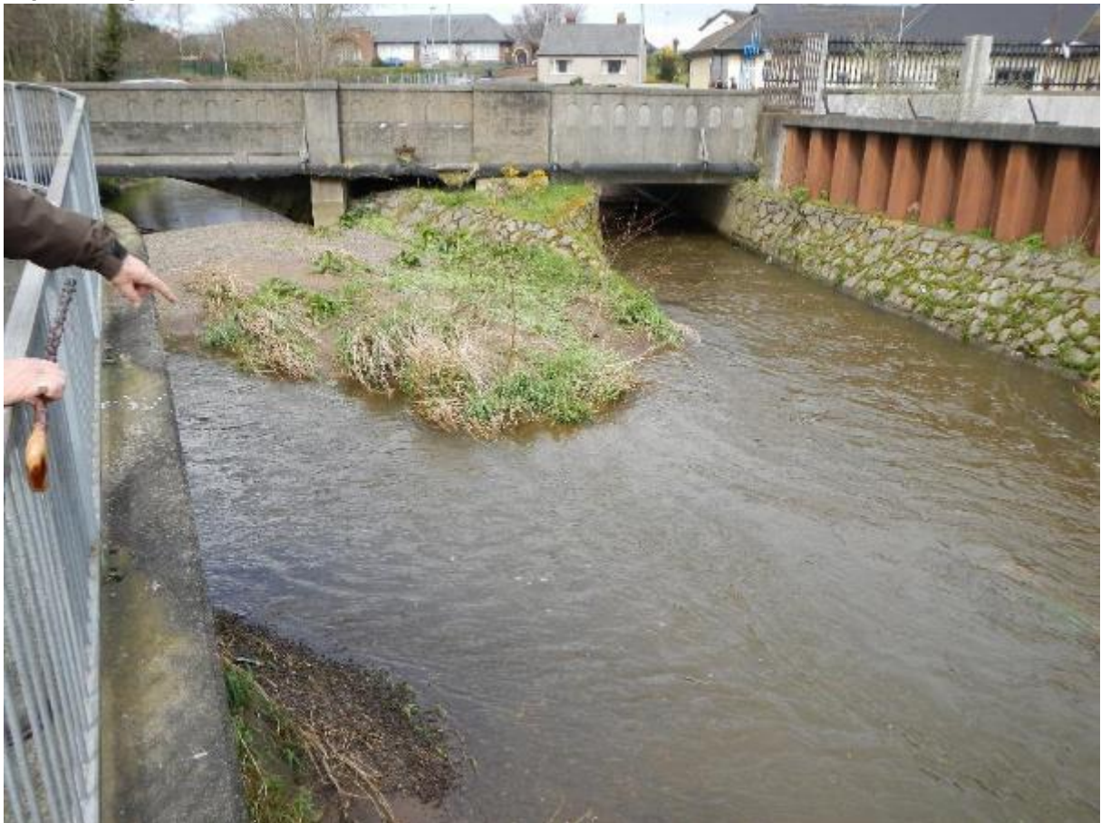
Figure 9. Deposition around the Newtownards Bridge. Removing this will simply reinstate the over-wide channel and result in more deposition. This work may be undertaken by the council to maintain capacity but would be of no real benefit to angling as it may even remove spawning gravels.
